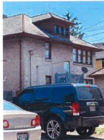
West roof facet.
