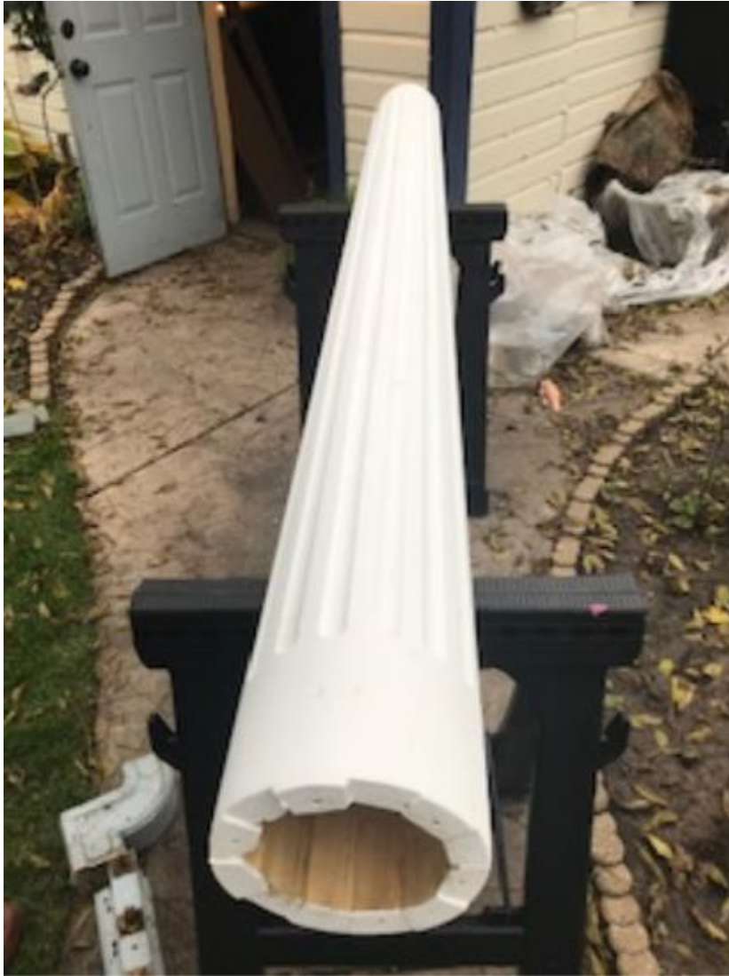
Photographs of the approved fluted cedar columns (columns were already painted and ready for installation at the time of photograph)
