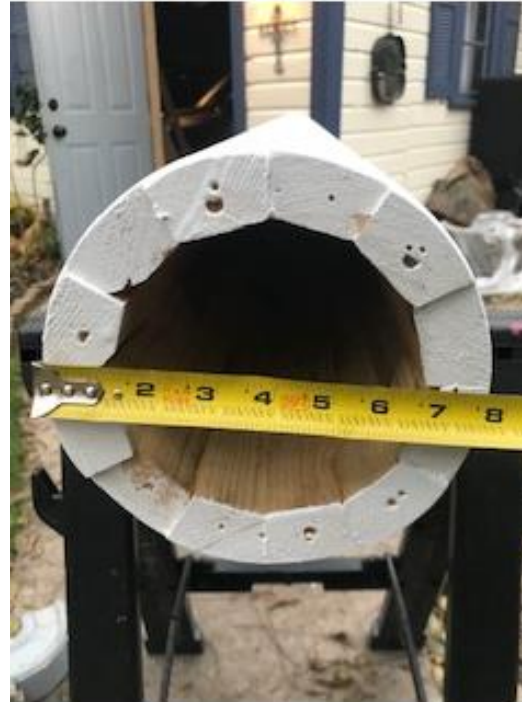
Photographs of the approved fluted cedar columns (columns were already painted and ready for installation at the time of photograph)
