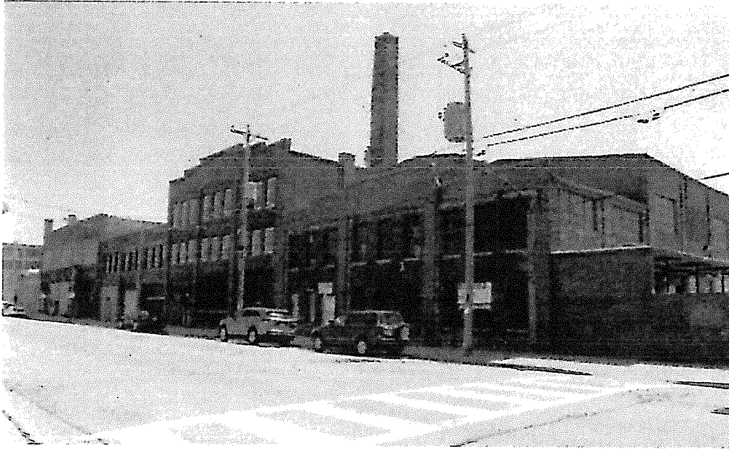
Figure 32. 1819-1739 W. St. Paul Avenue, view facing southeast.
