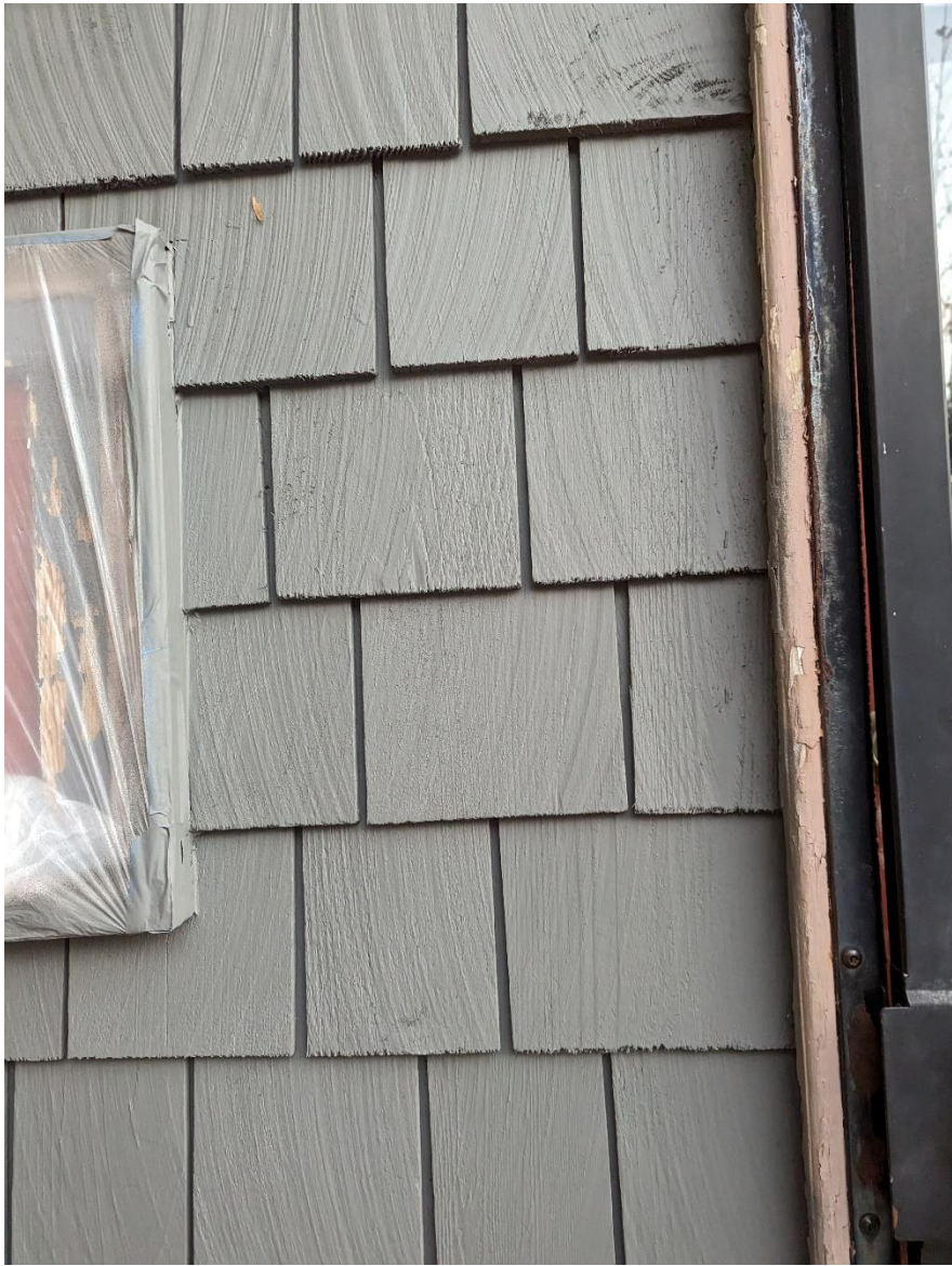
Replacement painted cedar shingles
