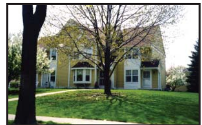
The first row house units built in the study area, on 42nd St. on land cleared for the Park West freeway; each of the three units shares party walls, yet has an individual entrance.
