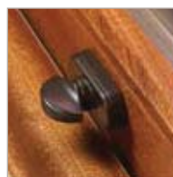
Turn knob lock on the bottom rail of the bottom sash in the closed position
