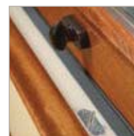
Turn knob and locking pin on the bottom of the bottom sash in the open position
