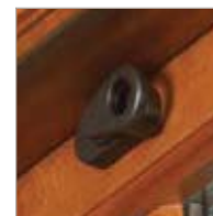
Heavy duty locking hardware on the top rail of the top sash
