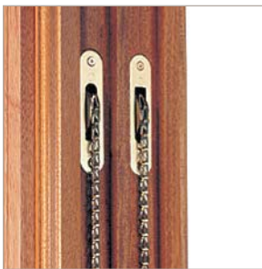
Brass chains and pulleys
