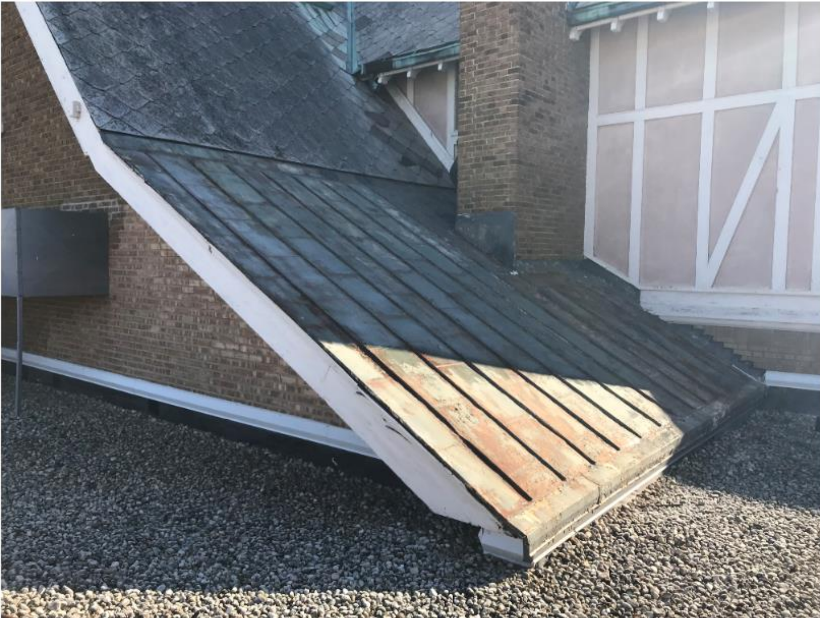
View of upper roof region to be repaired.
