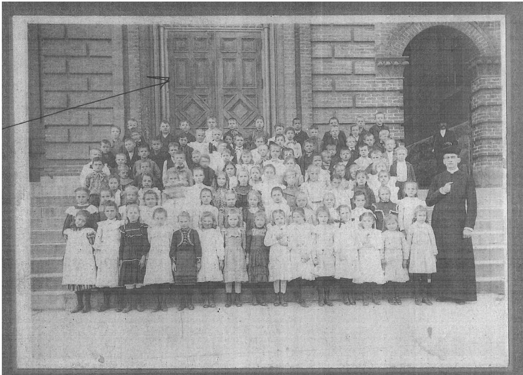
Historic doors shown in 1893 photograph.
