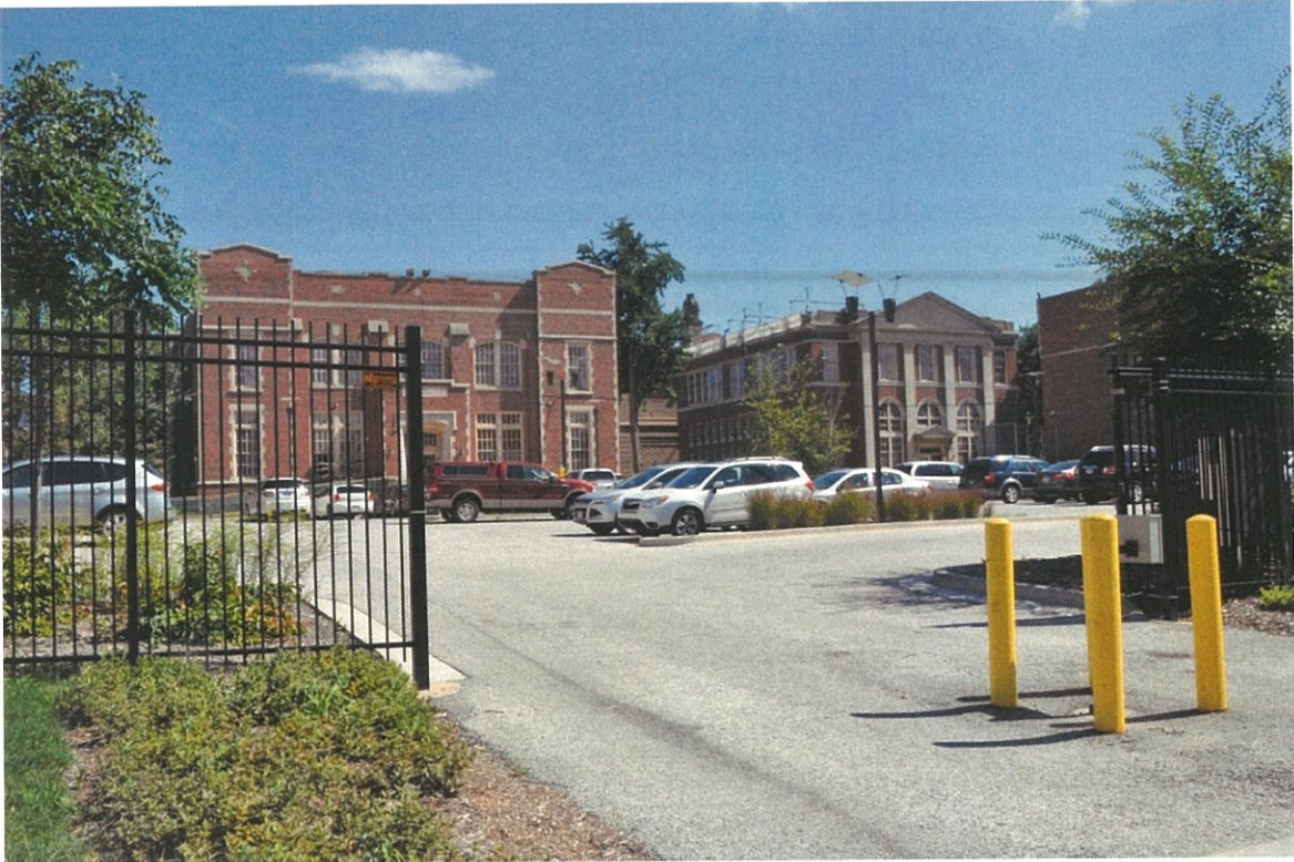
Photo 3 – View South East from 33rd
