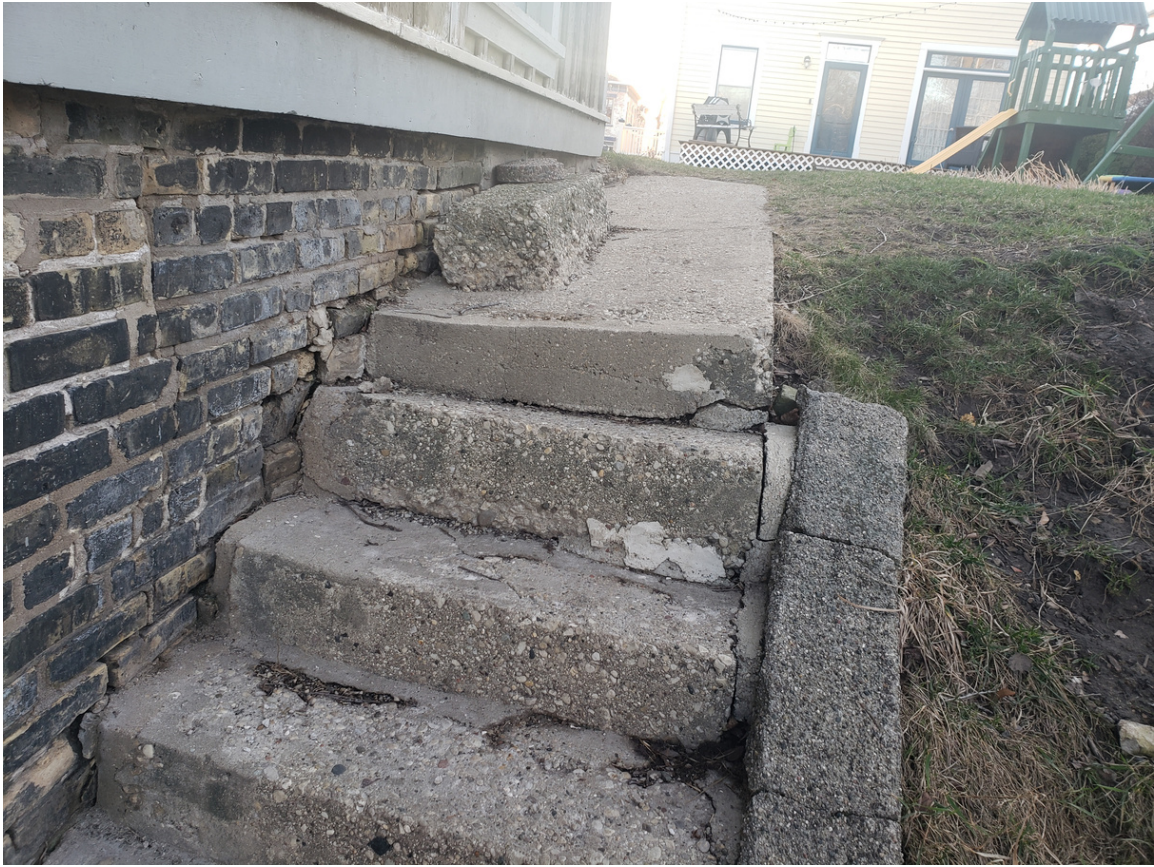
Existing stairs & damage to barn foundation
