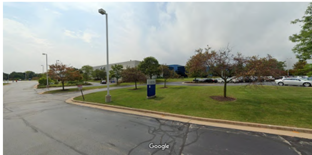
Northeast corner of existing building
