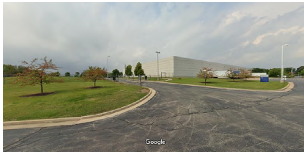
Southeast corner of existing building
