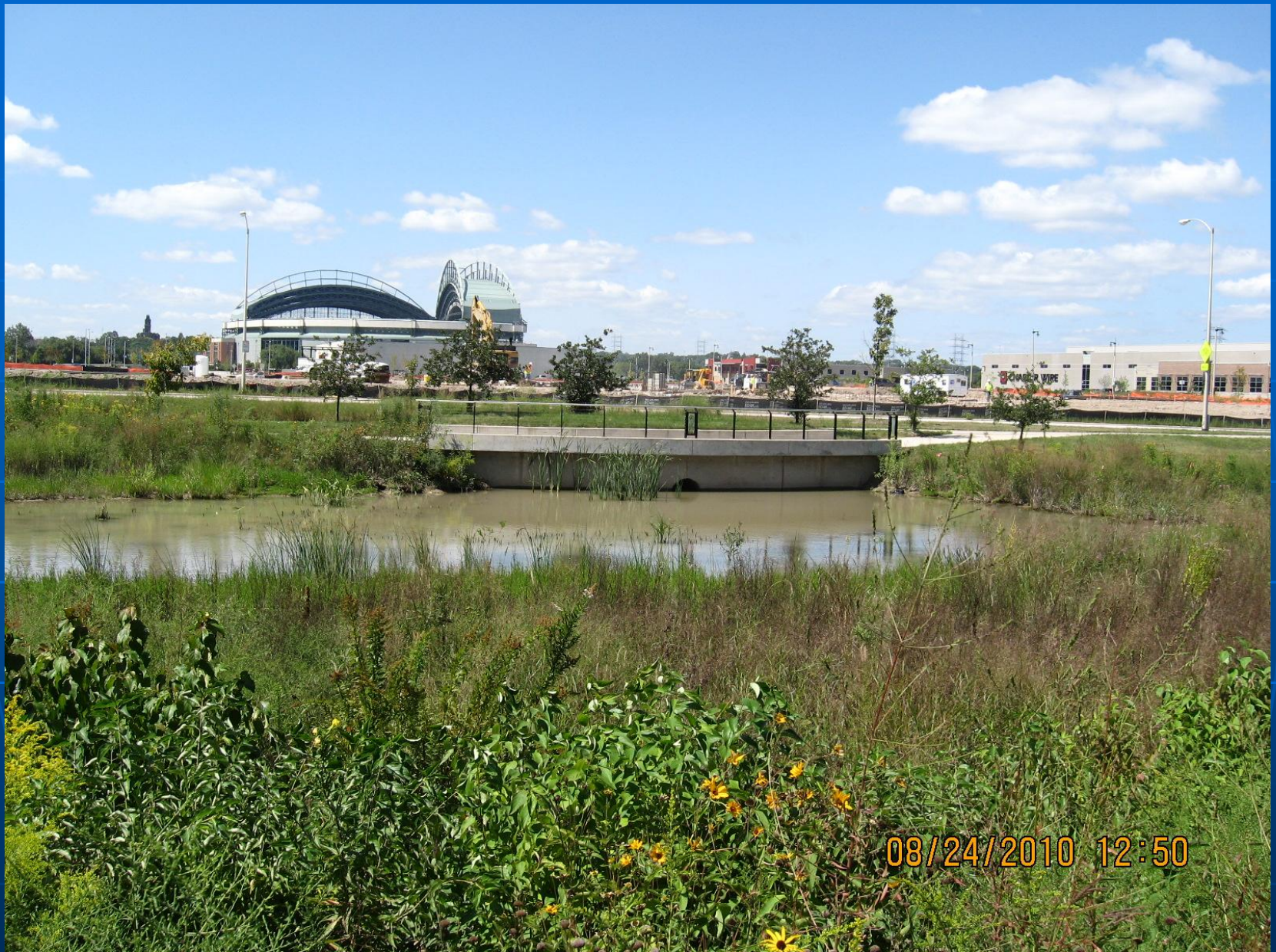
Bio-Retention Facility at 35 th and Canal
