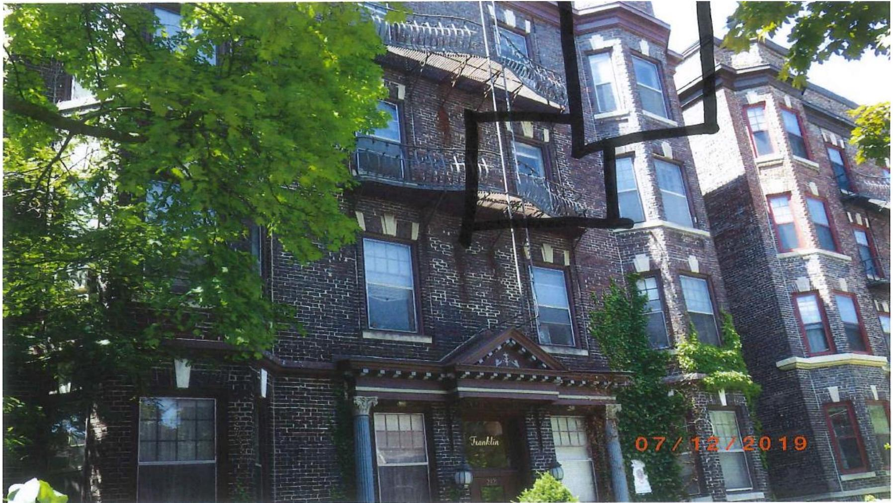
All three windows in the top floor bay indicated shall received new multi-pane sashes. The identified window on the third floor will receive the same.
