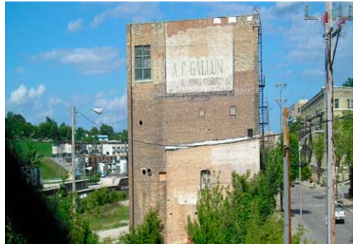
Figure 10.13: Industrial property along the river north of Holton Street.
