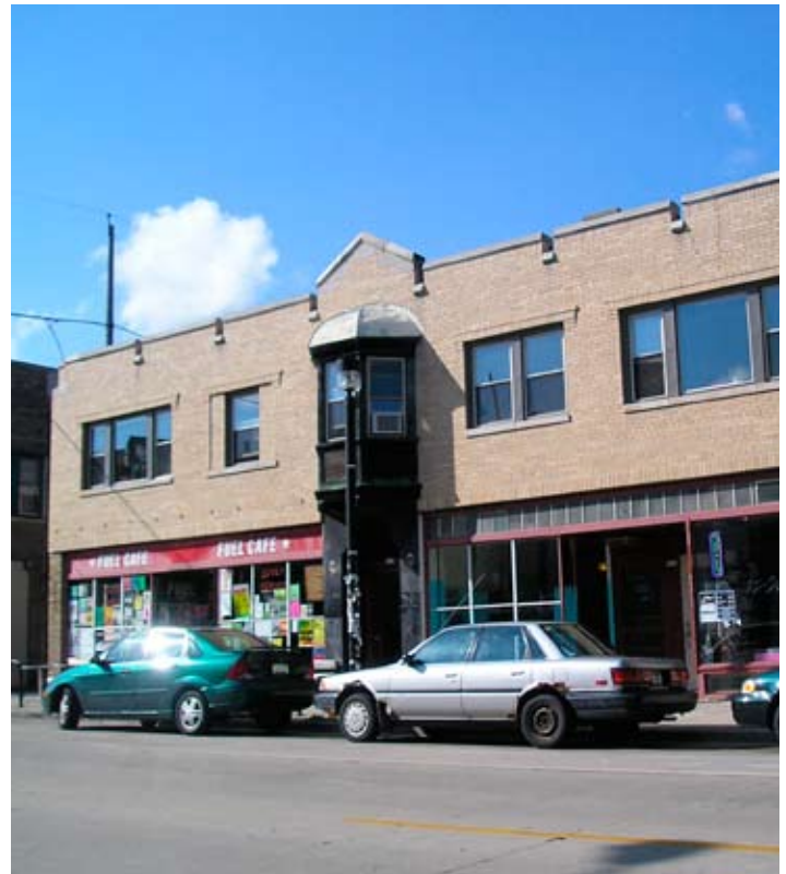
Figure 7.14: Center Street Commercial District
