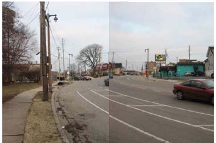
Figure 10.27: Approaching Brady Street from Water Street - Existing Conditions.
