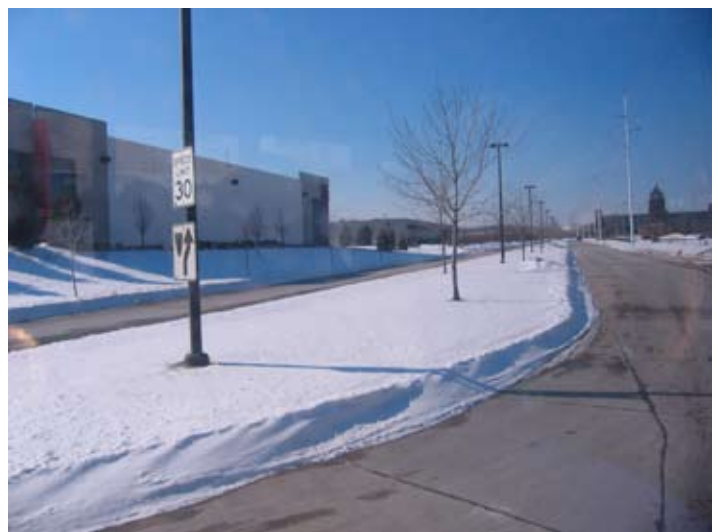
Figures 2.31 - 2.33: Industrial Buildings in Riverworks
