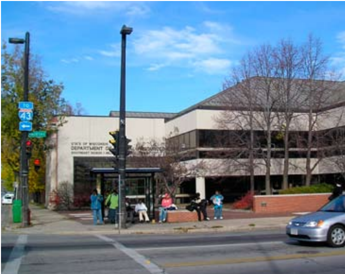
Figure 5.32: DNR Building and site to be Redeveloped
