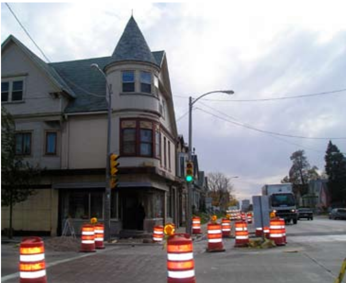
Figure 7.21: Holton Street - Existing Streetscape Conditions
