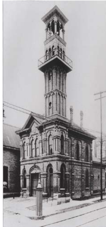
Figure 1.26: Historic Photo of the Brady Street Fire Station
