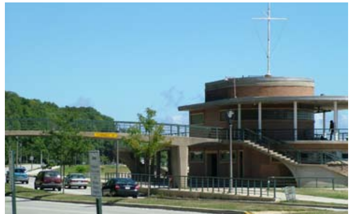
Figure 11.3: Pedestrian Bridge and Pavilion at Bradford Beach
