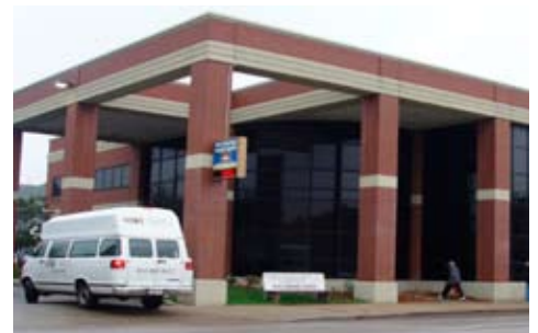
Figure 5.26: Heritage Health Center
