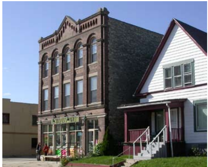
Figure 1.11: Holton Street mixed-use building
