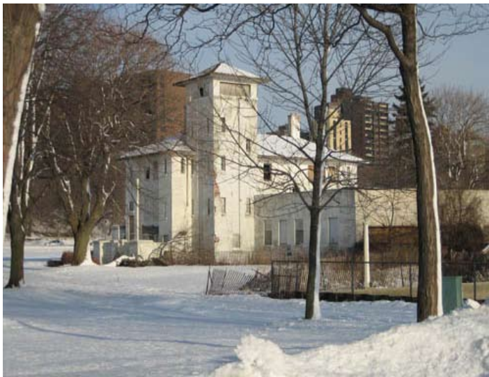
Figure 11.33: Former Coast Guard Station Slated for Demolition
