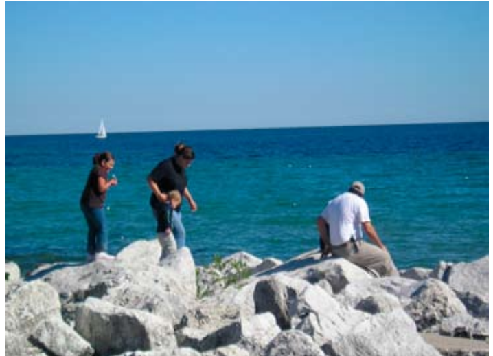
Figure 11.12: Riprap at McKinley Park preserves the shoreline and prevents erosion.
