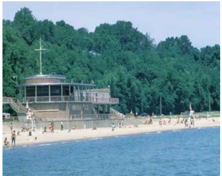
Figure 1.30: Bradford Beach with restored art deco beach house
