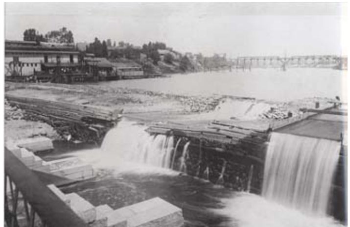
Figure 1.16: North Avenue Dam - Historic Photo
