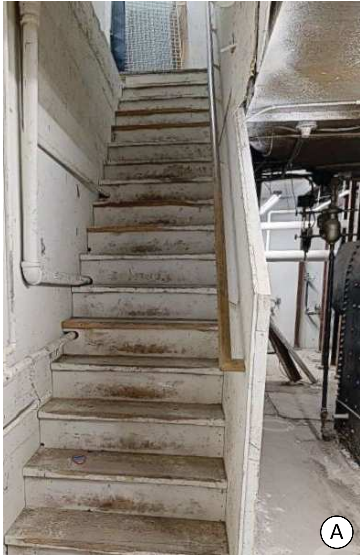
Staircase from first floor
