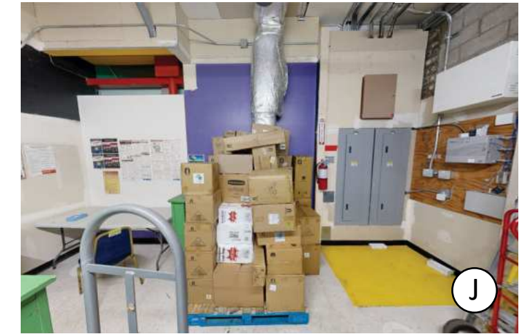
Back of Storage Room
