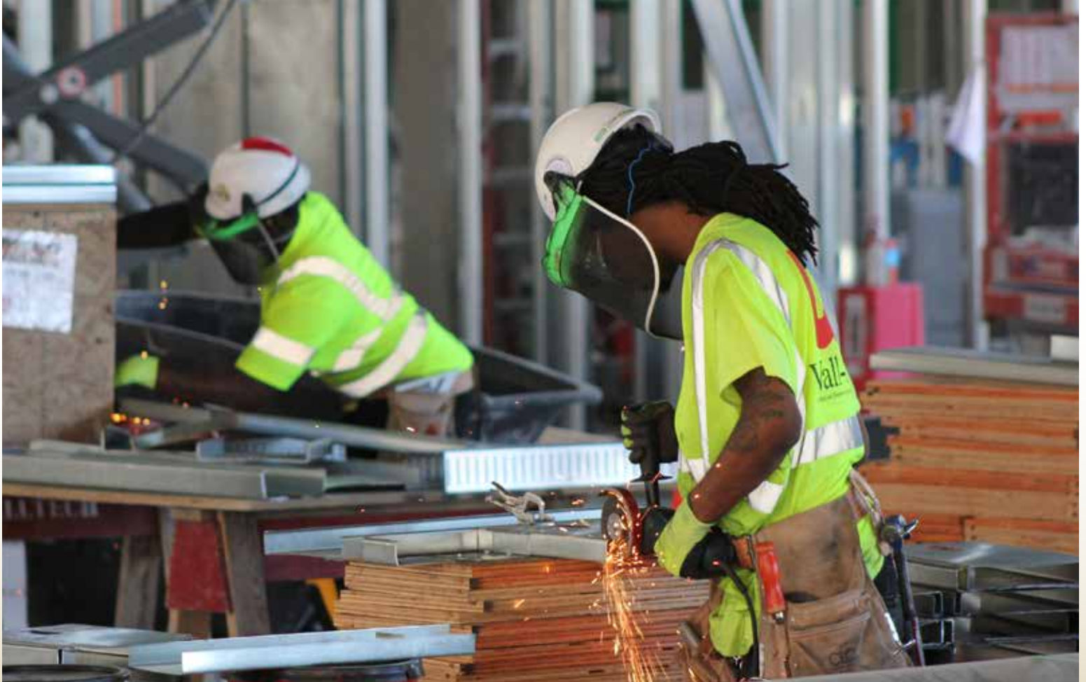
Carpenter working on the Milwaukee Arena site.
