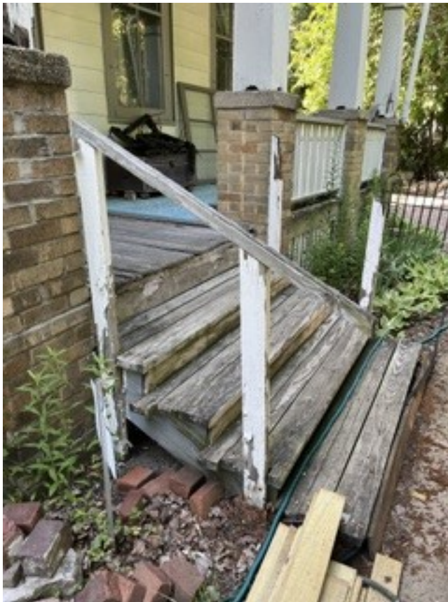
Existing handrails to be removed
