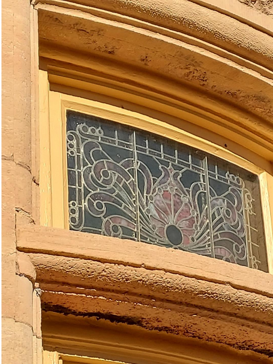
Photo Of Existing Storm Windows (New will match these)
