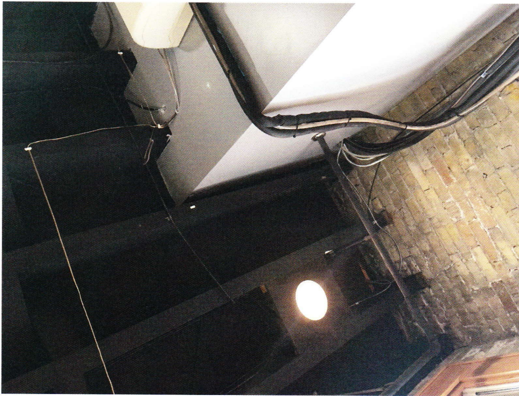
INSIDE BUILDING IN OPEN JOIST SPACE
