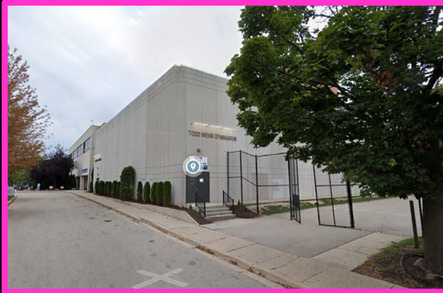
View from internal drive looking south-west
