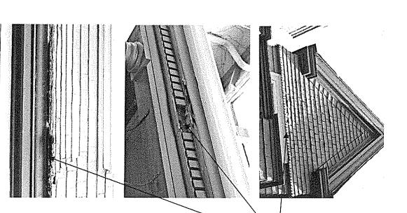
Spot replace damaged or deteriorated wood trim, sidewall shingling, dentil block and trim with matching new wood
