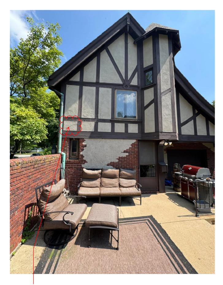
ADD 8" COPPER EXHAUST VENT WITHIN THIS STUCCO SECTION FOR RANGE HOOD.
