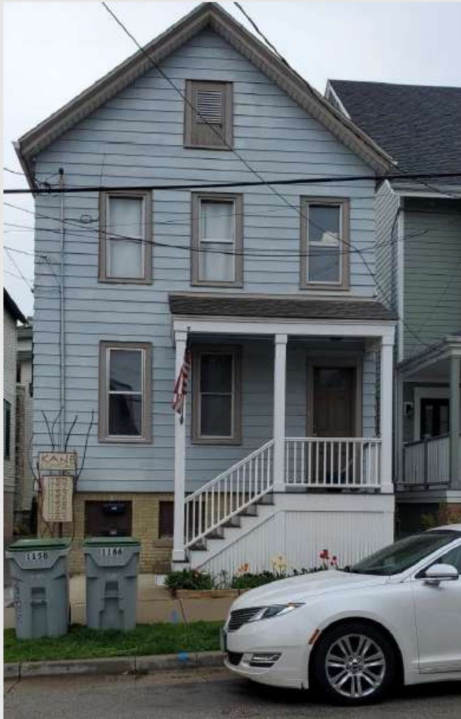
File Number 260047. Site Photos – Existing North and South Elevations.
