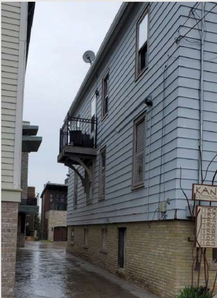
West Elevation looking North
