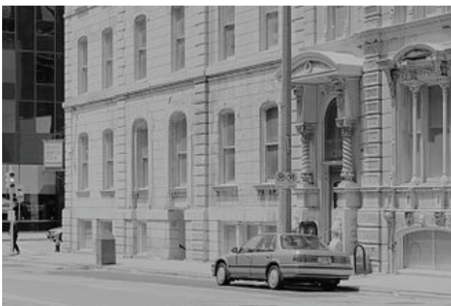
IMAGE 3: Detail of historic photograph ca. 1980s showing the current sign at the southwest corner (far left). © Milwaukee County Historical Society.
