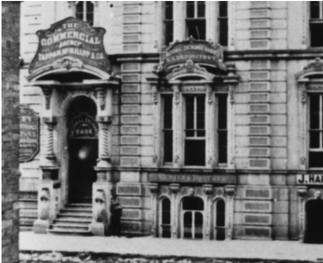
IMAGE 1: Historic photograph dated ca. 1865-1876 showing the entrance at 210 E. Michigan entrance with no door design details visible. © Milwaukee County Historical Society.
