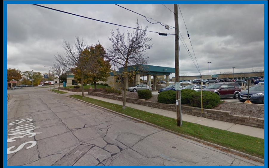
View from South 34 th Street looking north-east
