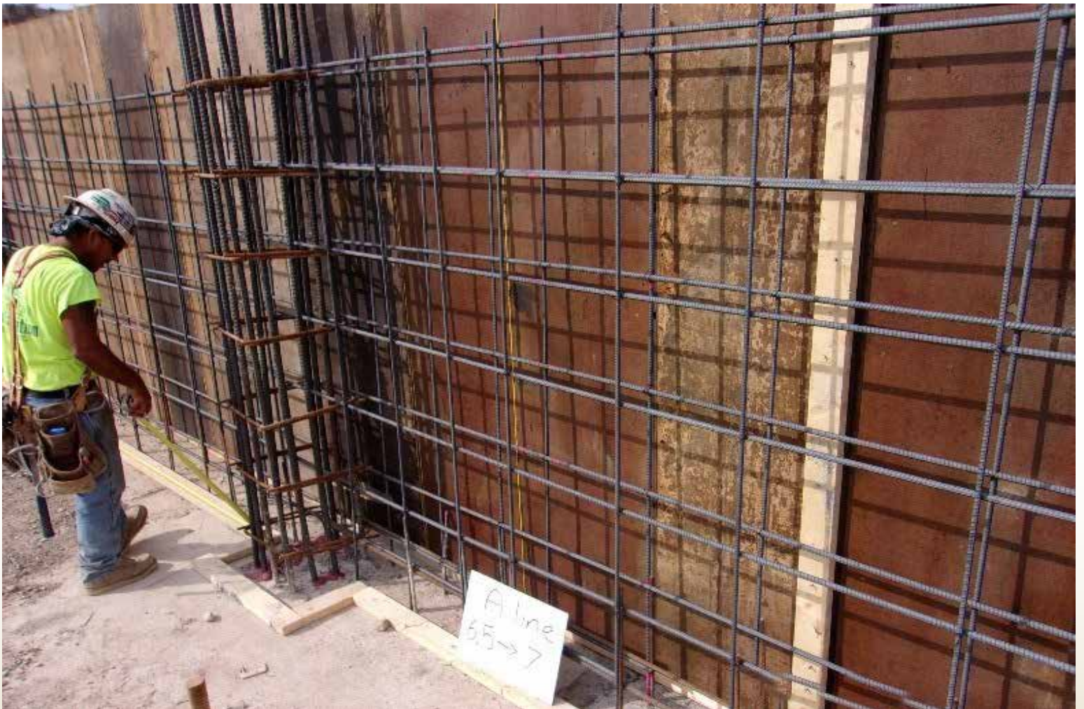
Photo of Grid Line A Foundation Wall
