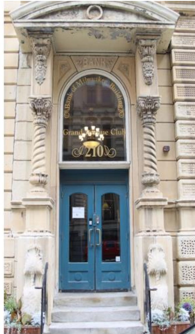
EXISTING ENTRY LOCATION (SOUTH ELEVATION)
