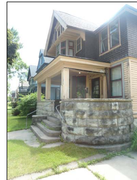
LOOKING SOUTH WEST
