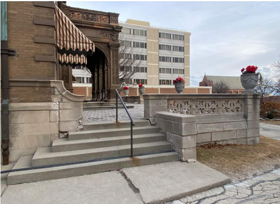
Photo 12: West Side of South Entrance Terrace Showing Stone & Paver Deterioration
