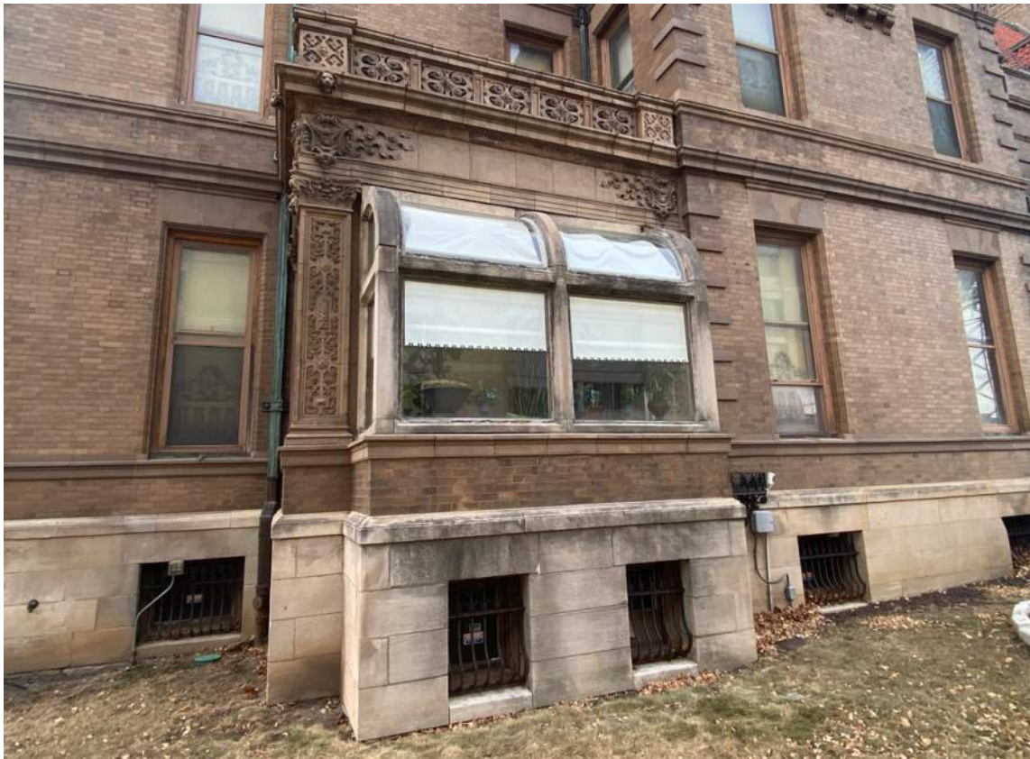
Photo 06: Detail of Conservatory. Non-original stone window framing to be removed and replaced with new to match original.
