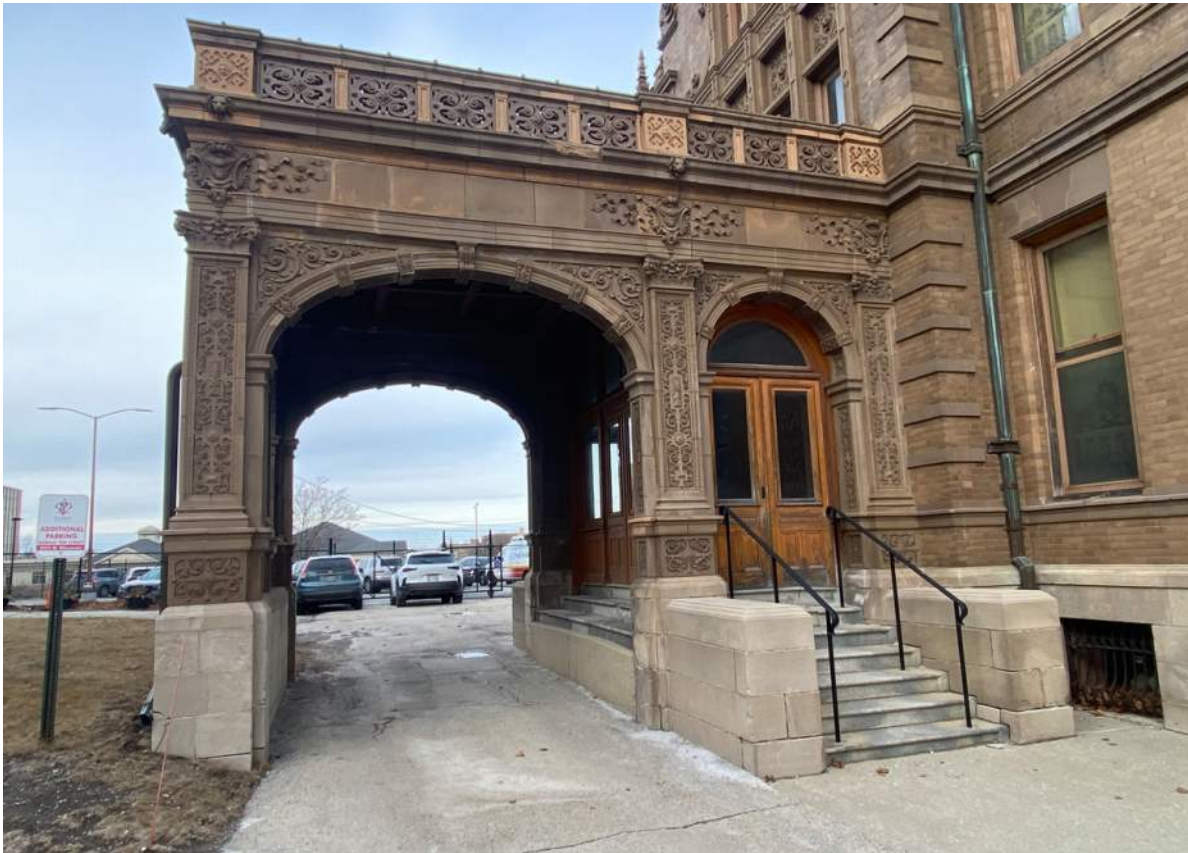
Photo 03: South View of Porte Cochere showing drop in terra cotta arch stones and deterioration of entry steps.
