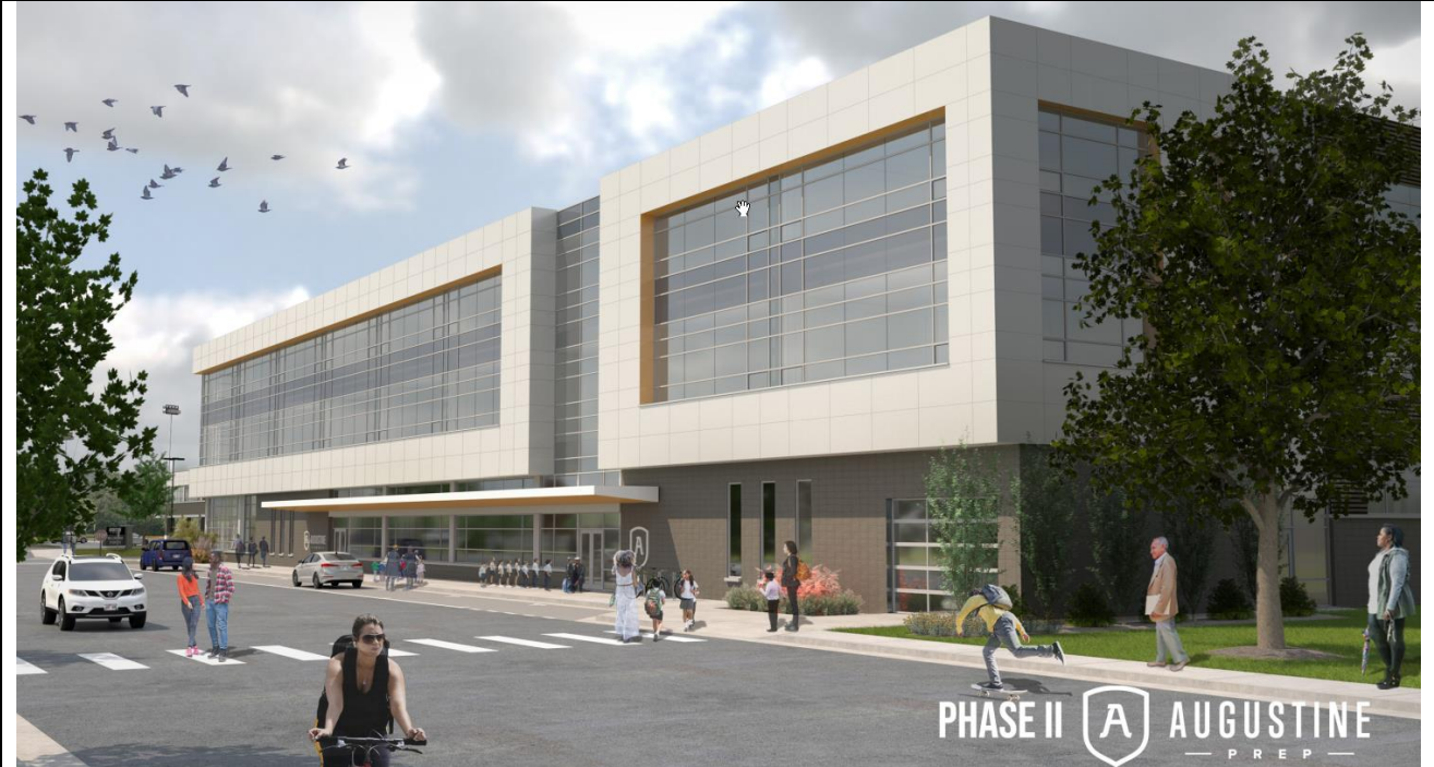
View to Main Façade on South 5th Street
