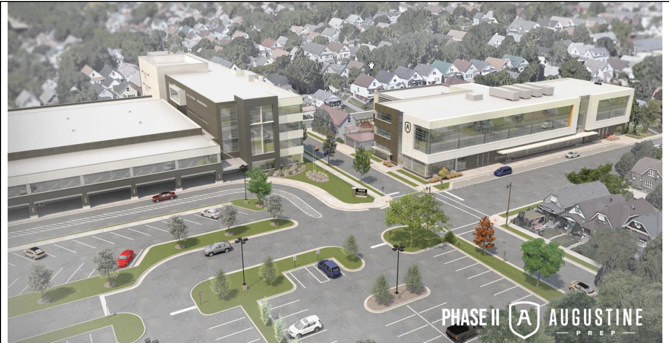
Aerial View to the Northwest.
