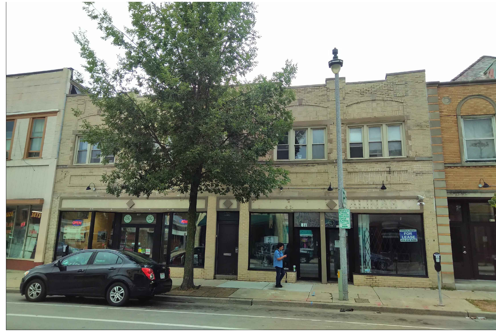
EXISTING NORTH FACADE; ALUMINUM STOREFRONT IS ABOUT 20 YEARS OLD ALONG WITH THE EIFS BANDING.
