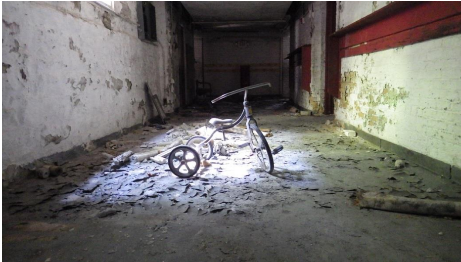
Interior hallway photo, 2001 West Vliet Street
