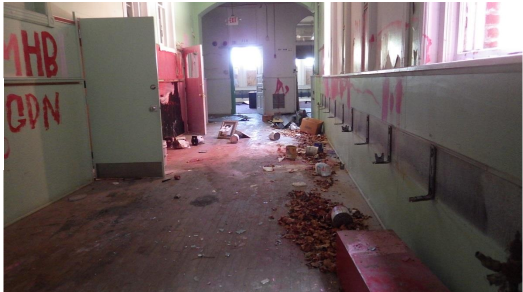
Interior hallway, 2001 West Vliet Street
