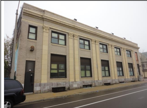
Looking southeasterly from N. Holton Street
