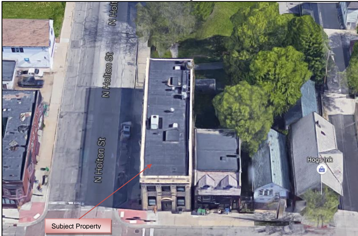
View Looking North
