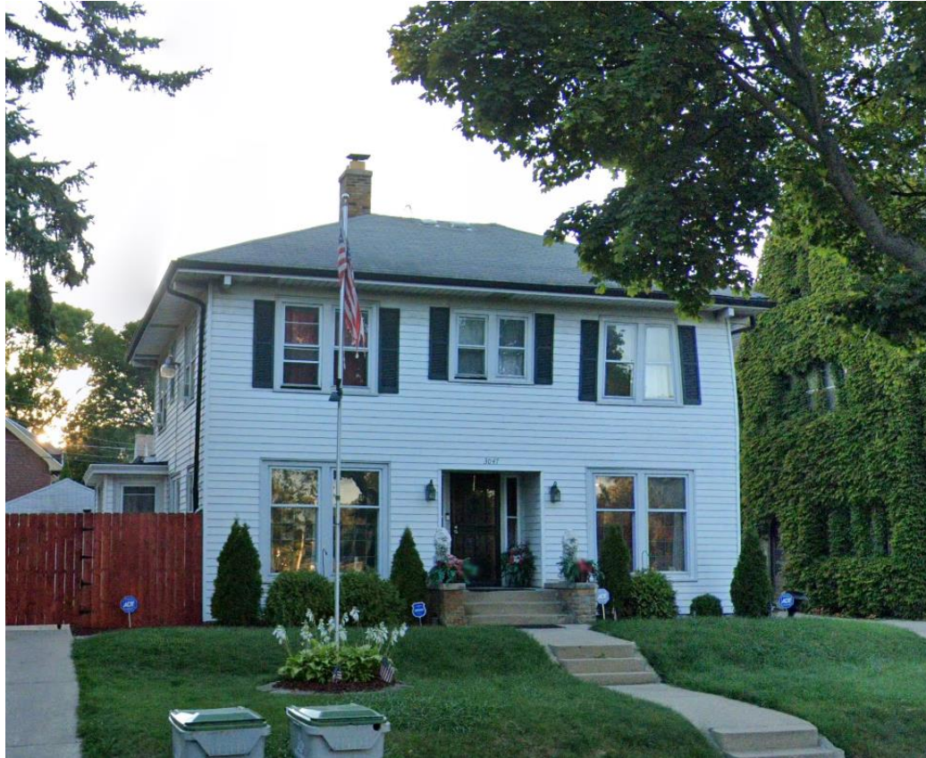
Current house conditions and approved shingle.
