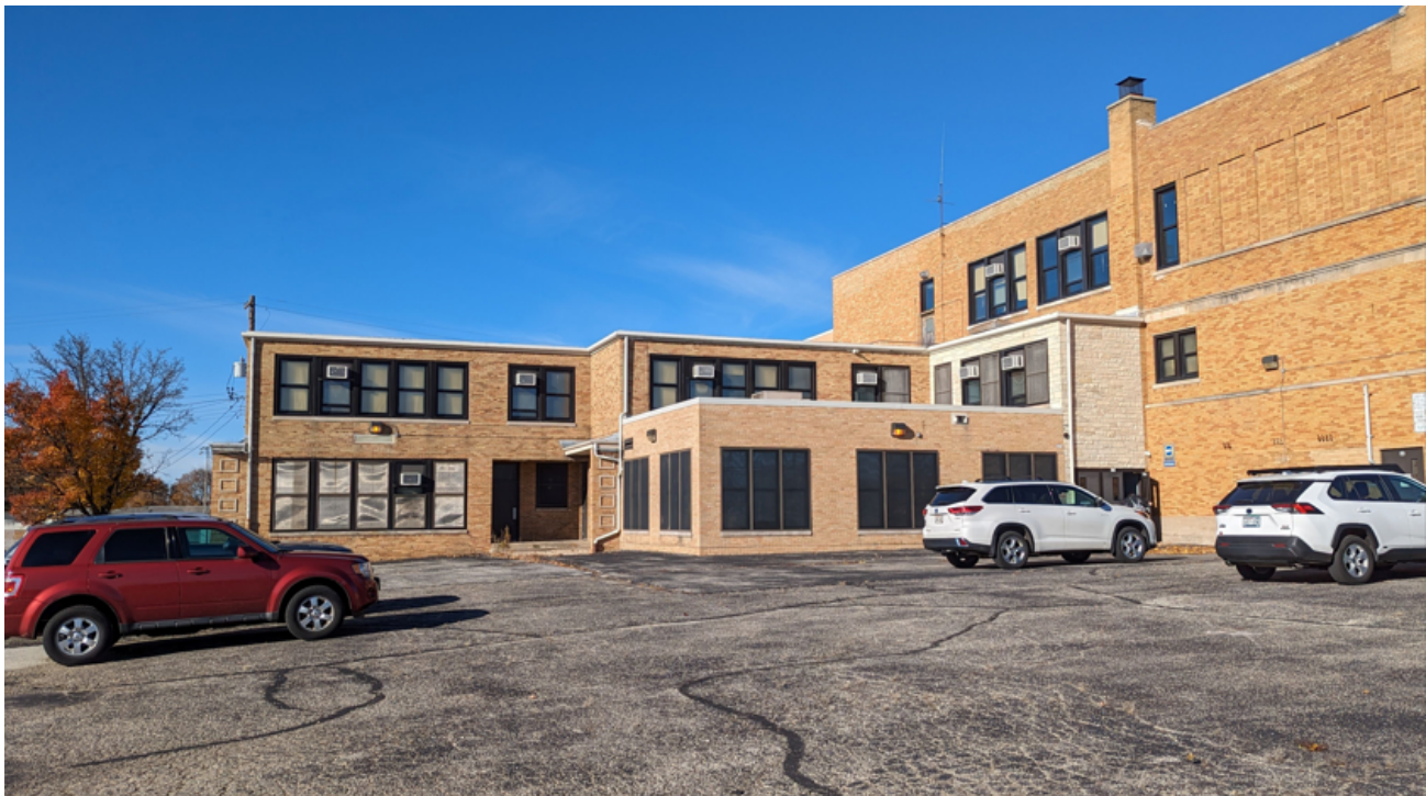
Photo 8 - East Elevation - 1954 & 1999 Building (portions of South Elevation of 1929, 1937, & 1943 Building visible)
