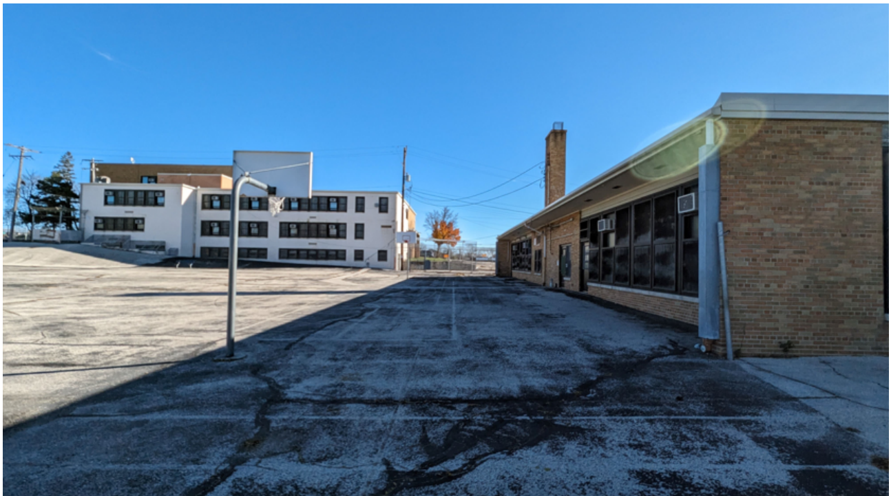
Photo 4 - Main West Elevation - 1954 Building & Northwest Elevation - 1951 Building
