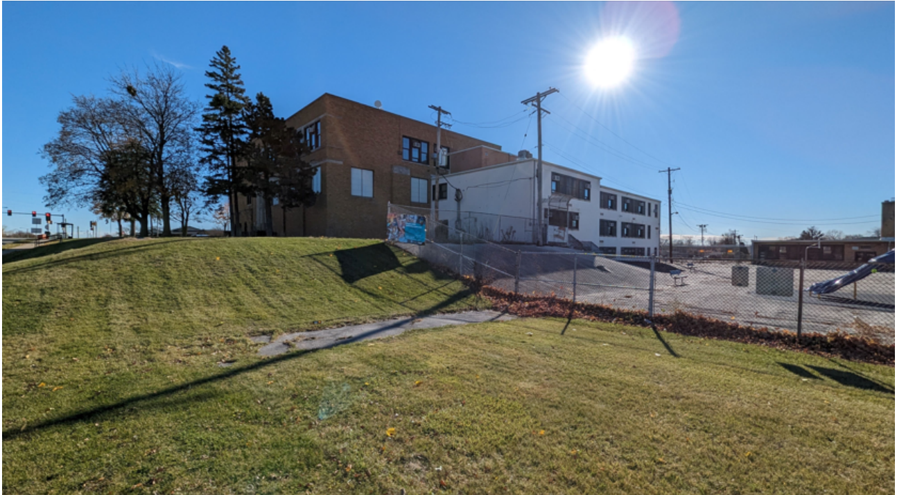
Photo 3 - Northwest Elevation - 1943 & 1954 Buidling
