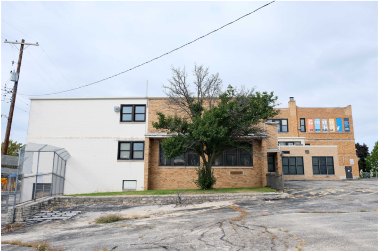
Photo 7 - South Elevation - 1954 & 1999 Building (1929, 1937, & 1943 portions visible in background)
