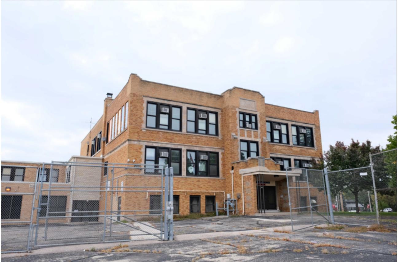
Photo 1 - East Elevation - 1929 & 1937 Building to be adaptively reused
