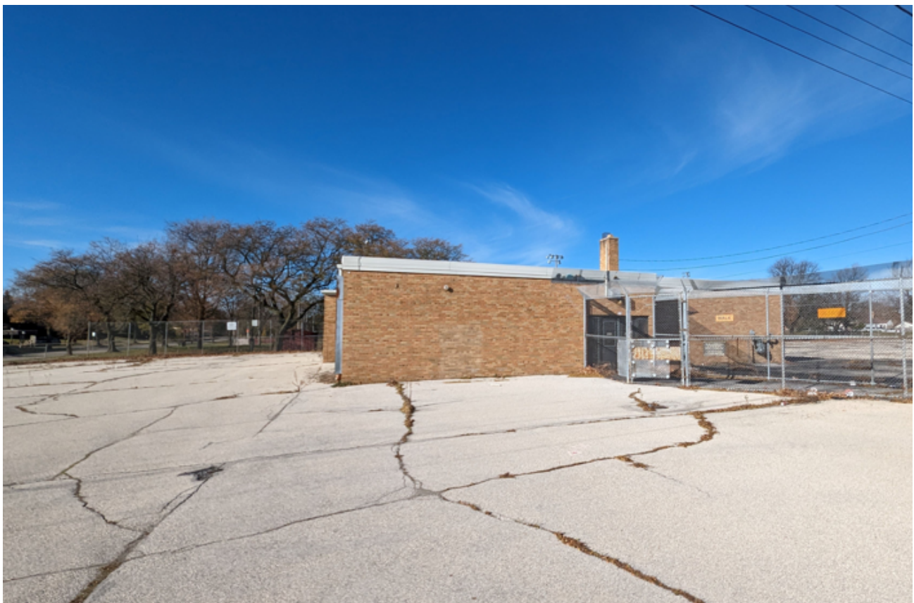
Photo 6 - East Elevation - 1951 Building
