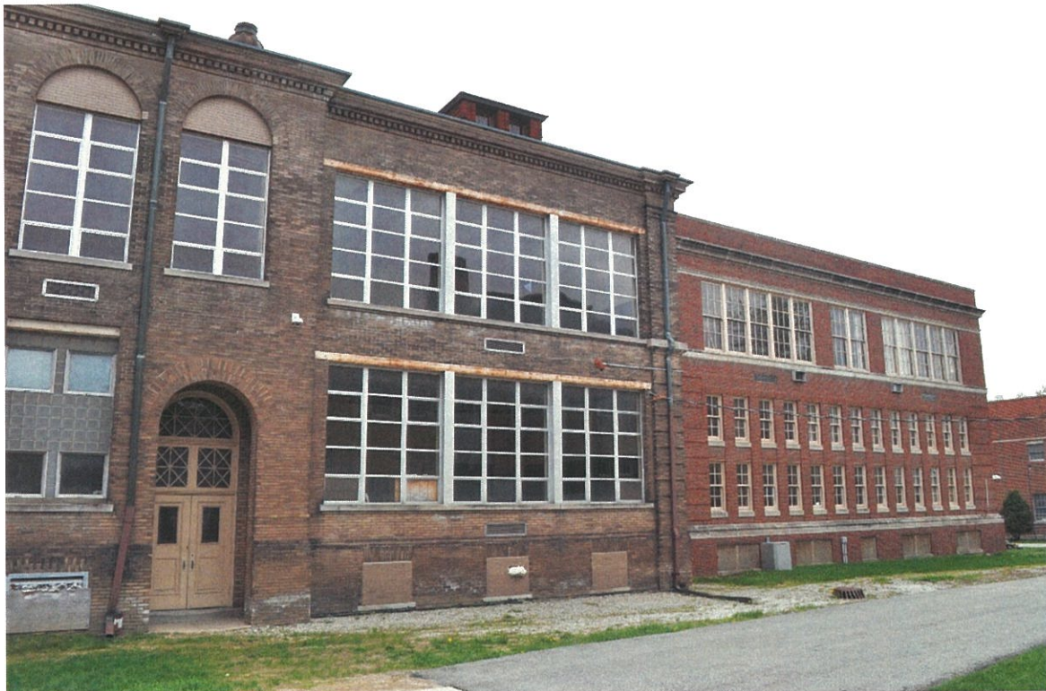
Photo 6 - North elevation of Albrecht Hall and Library
