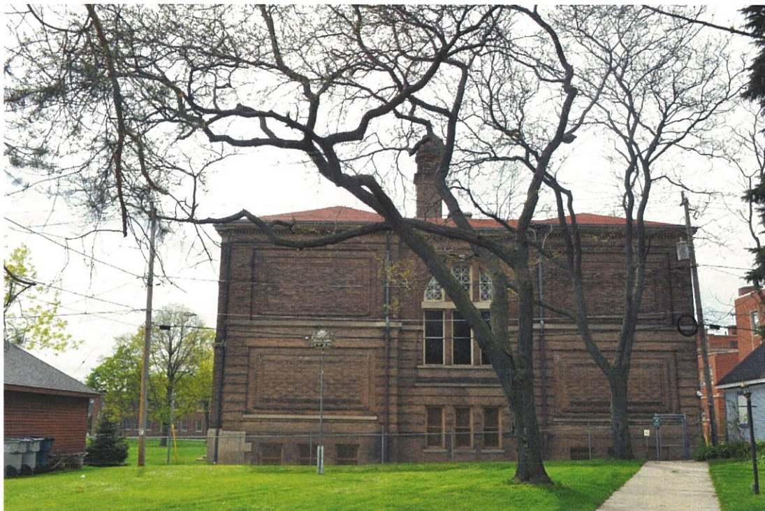
Photo 4 - East elevation of Albrecht Hall
