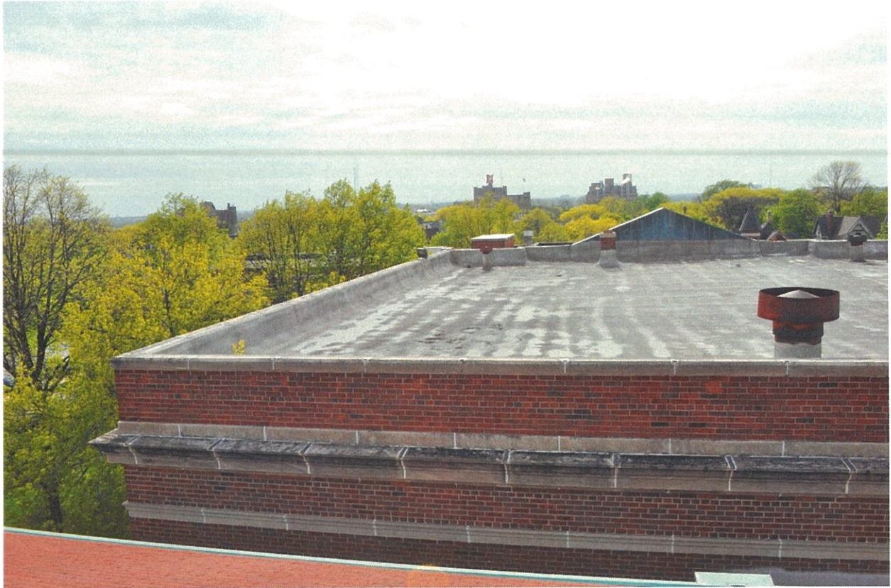
Photo 9 - Library Roof, looking west
