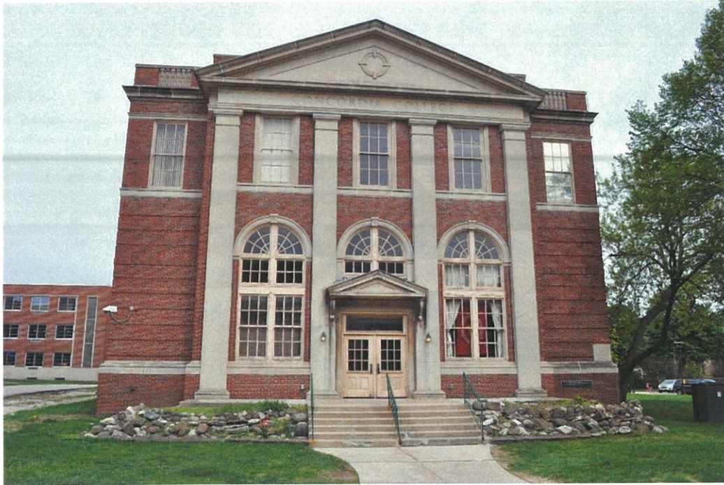
Photo 1 - West elevation of Library
