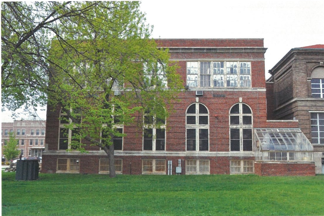
Photo 2 - South elevation of Library
