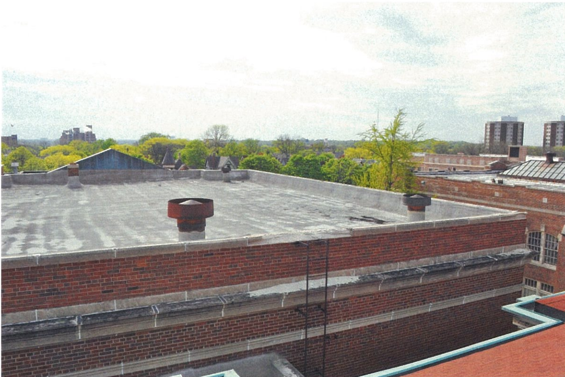
Photo 8 - Library Roof, looking northwest
