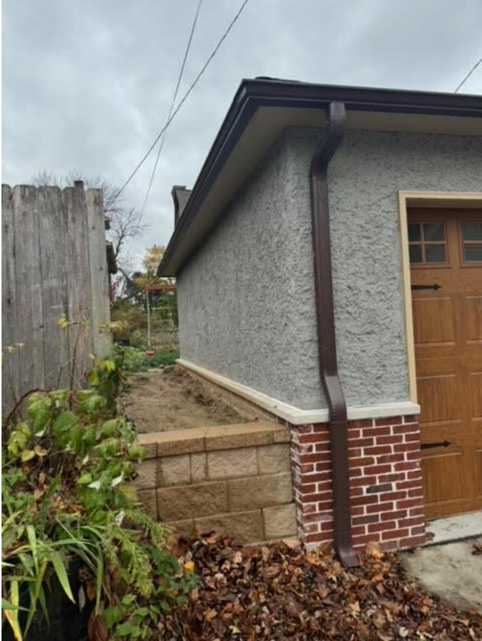
East Side Garage
