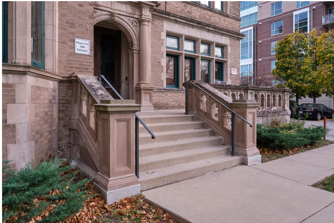
IMAGE 10: View of the existing entry terrace
