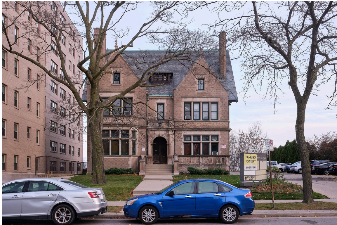
IMAGE 01: View from the west
