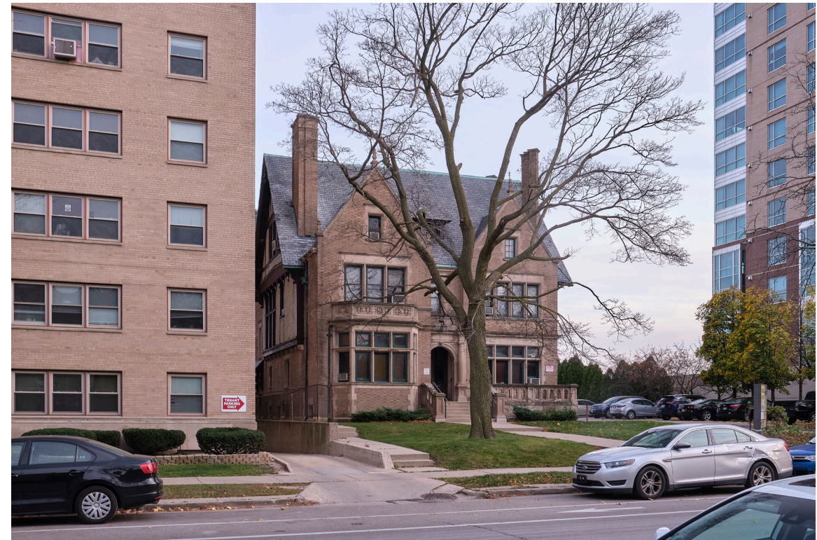
IMAGE 12: View from the northwest - opposite sidewalk
