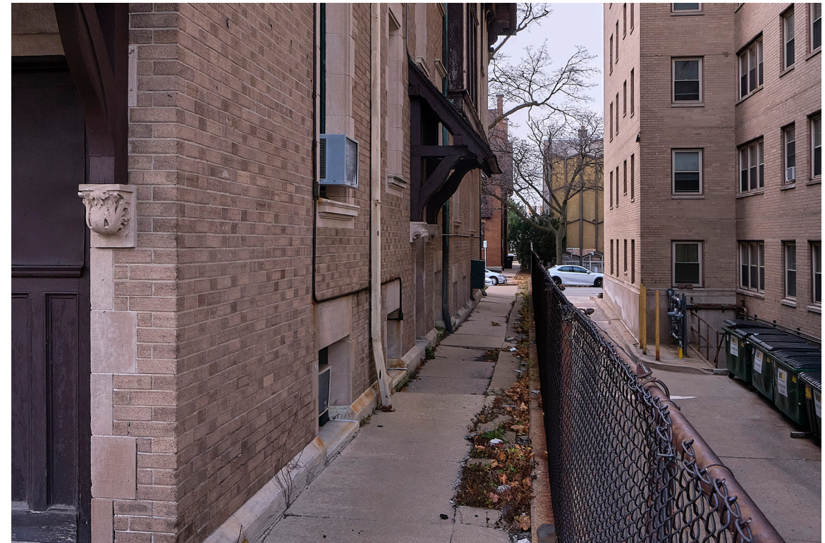
IMAGE 08: View from the northeast (lower)
