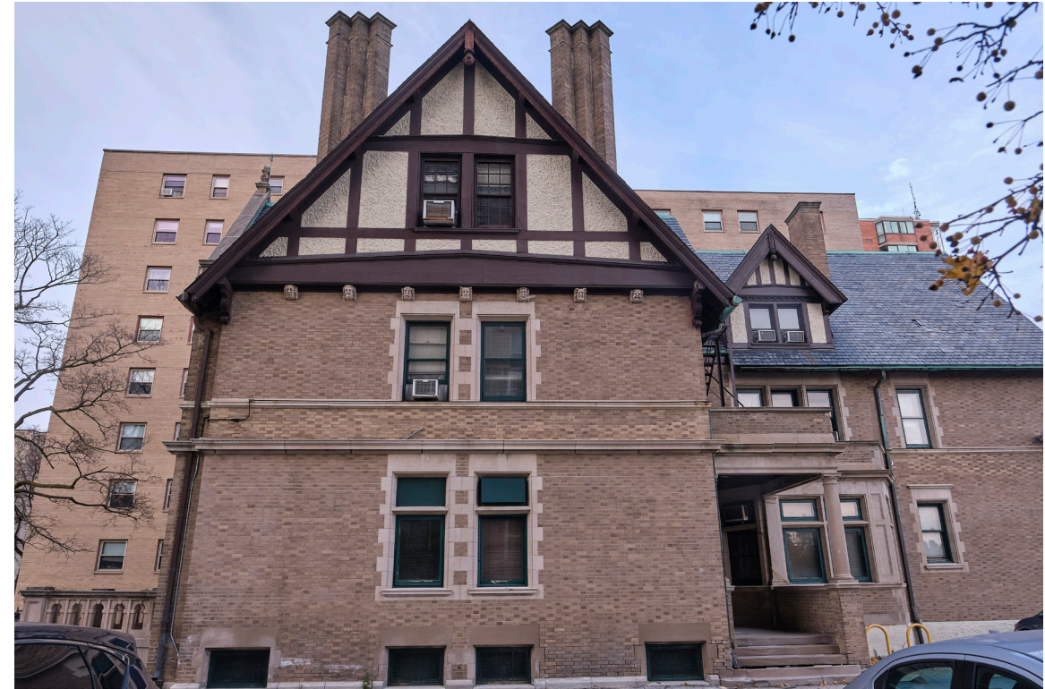
IMAGE 03: View from the south
