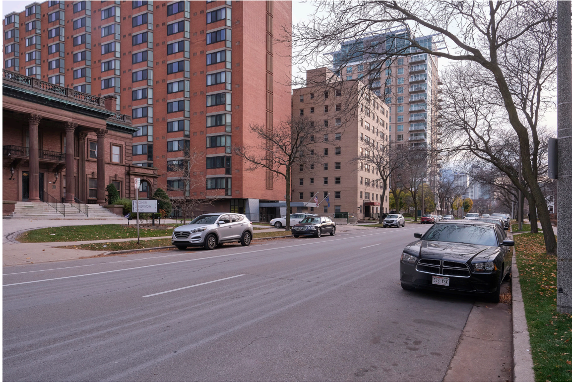
IMAGE 15: View from the northwest - opposite sidewalk
