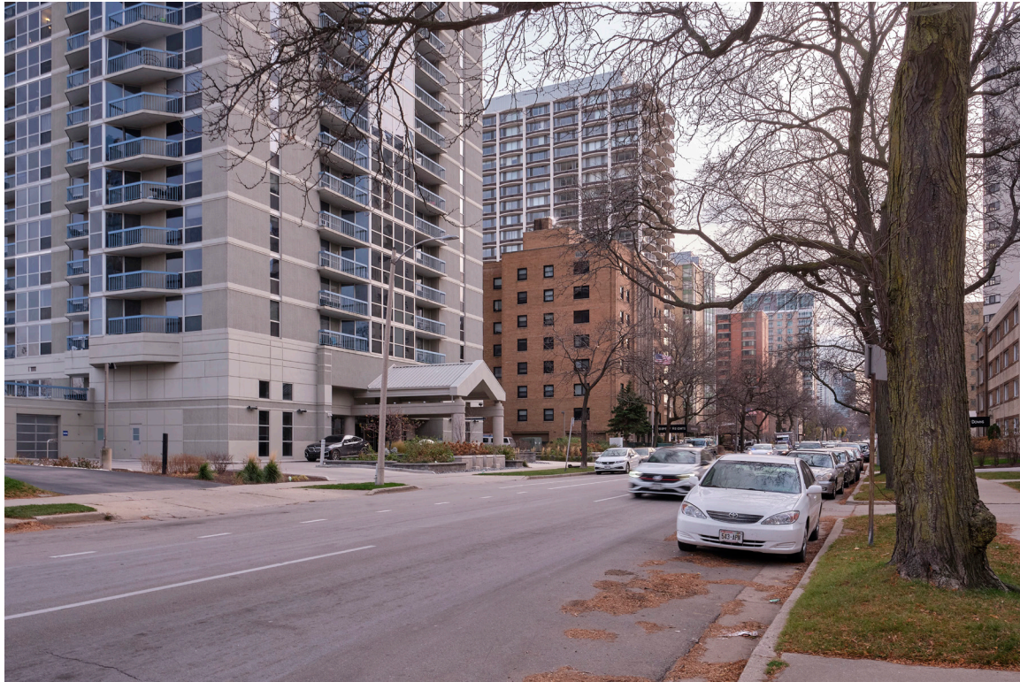
IMAGE 16: View from the northwest - opposite sidewalk
