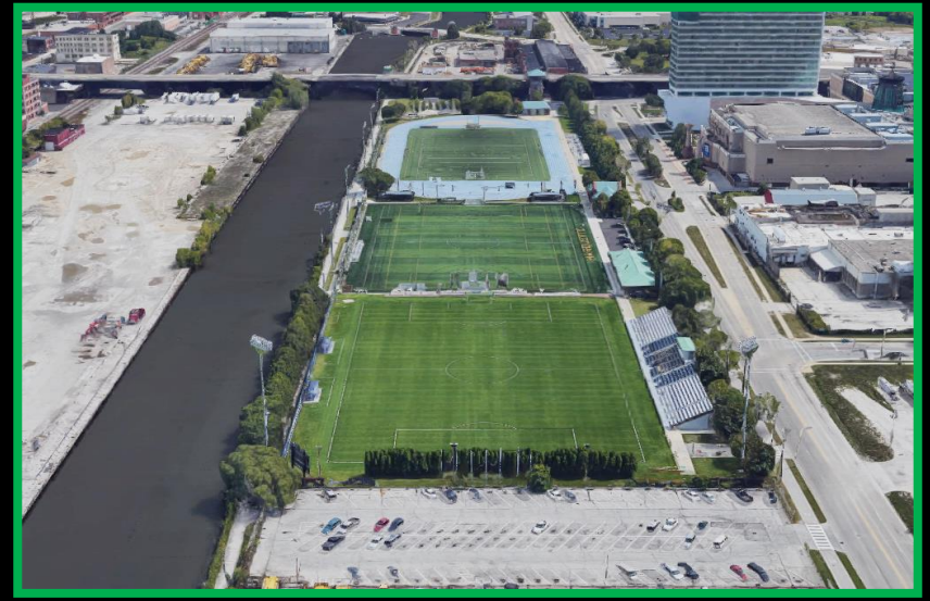
Aerial view looking east
