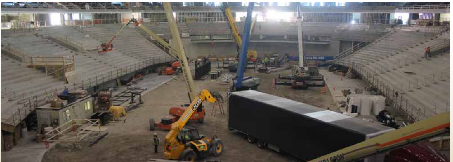
Interior construction of WESC.
