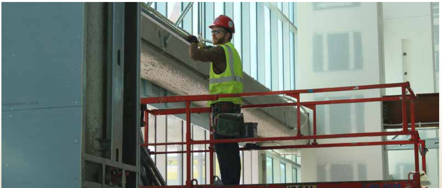
Carpenter working on the WESC.
