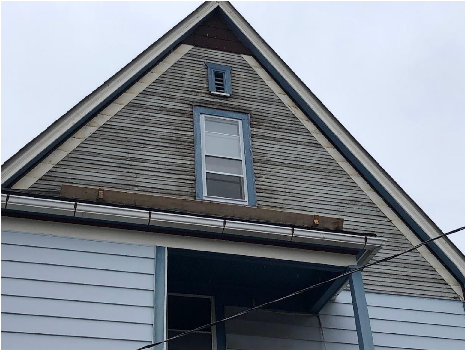
Clapboard in west facade
