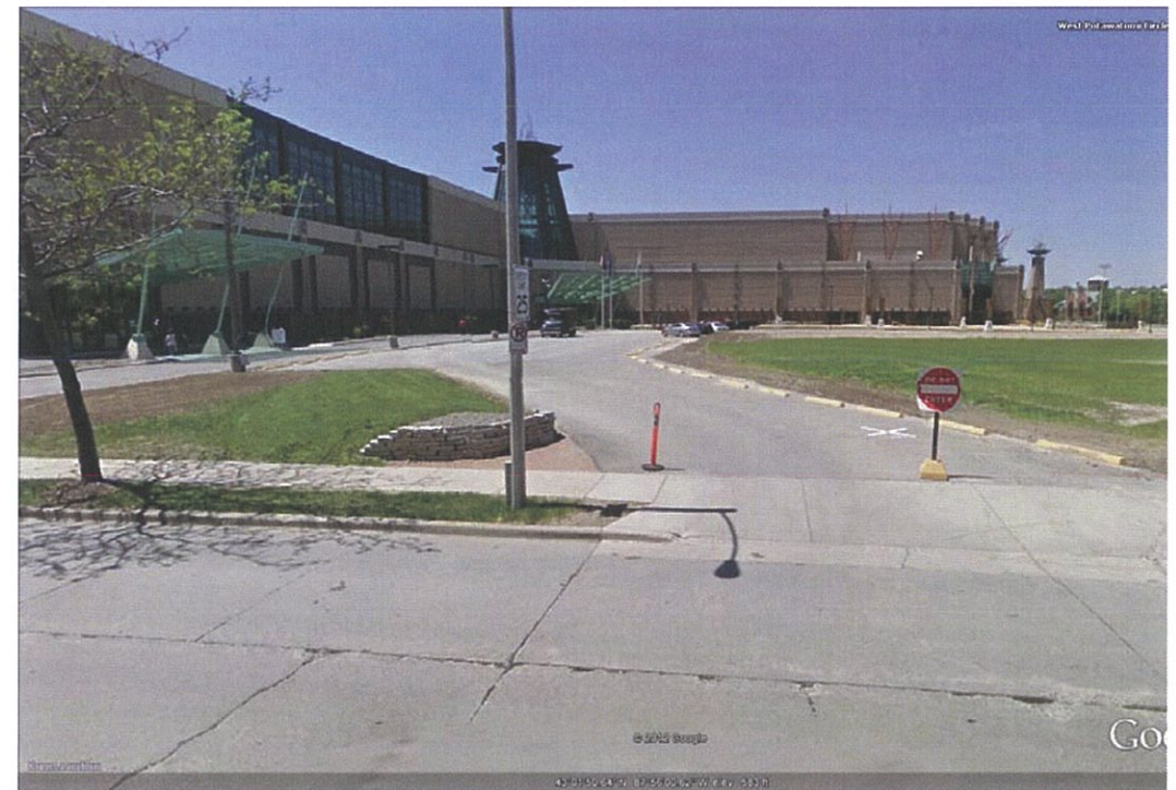
Looking westbound toward Casino at auxiliary exit driveway.
