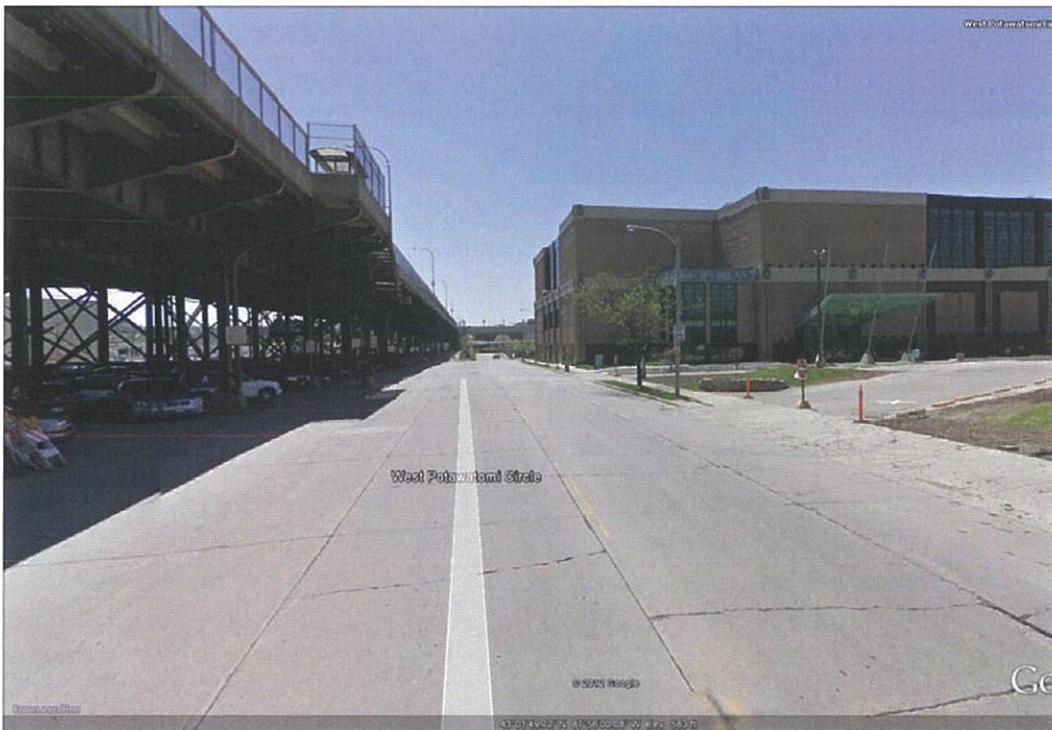
Looking southbound along Potawatomi Circle towards across Casino exit driveway.
