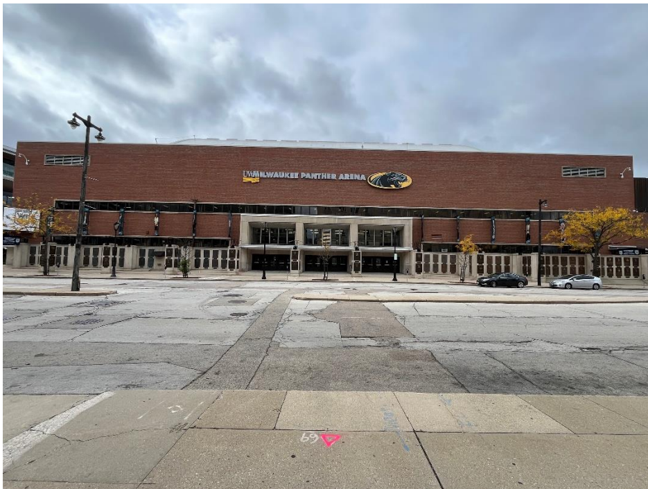
Figure 22 East façade of the Arena, 2025.
