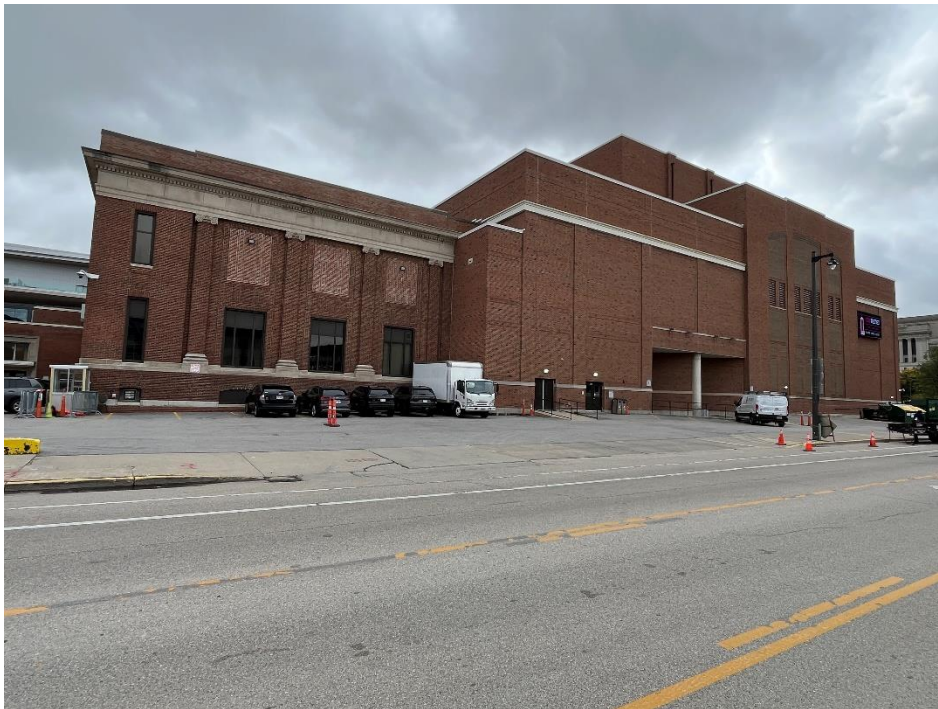
Figure 16 North façade of the Auditorium, 2025.
