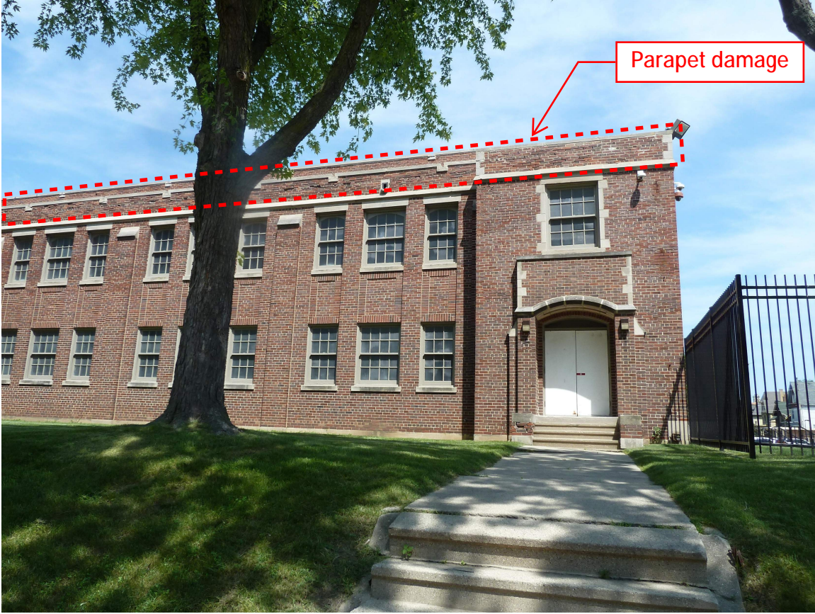
Photo 12 - West (southern portion) at Gymnasium
