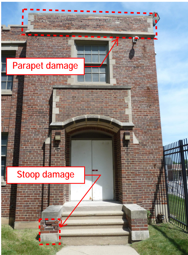
Photo 15 - West Entry (southern portion) at Gymnasium
