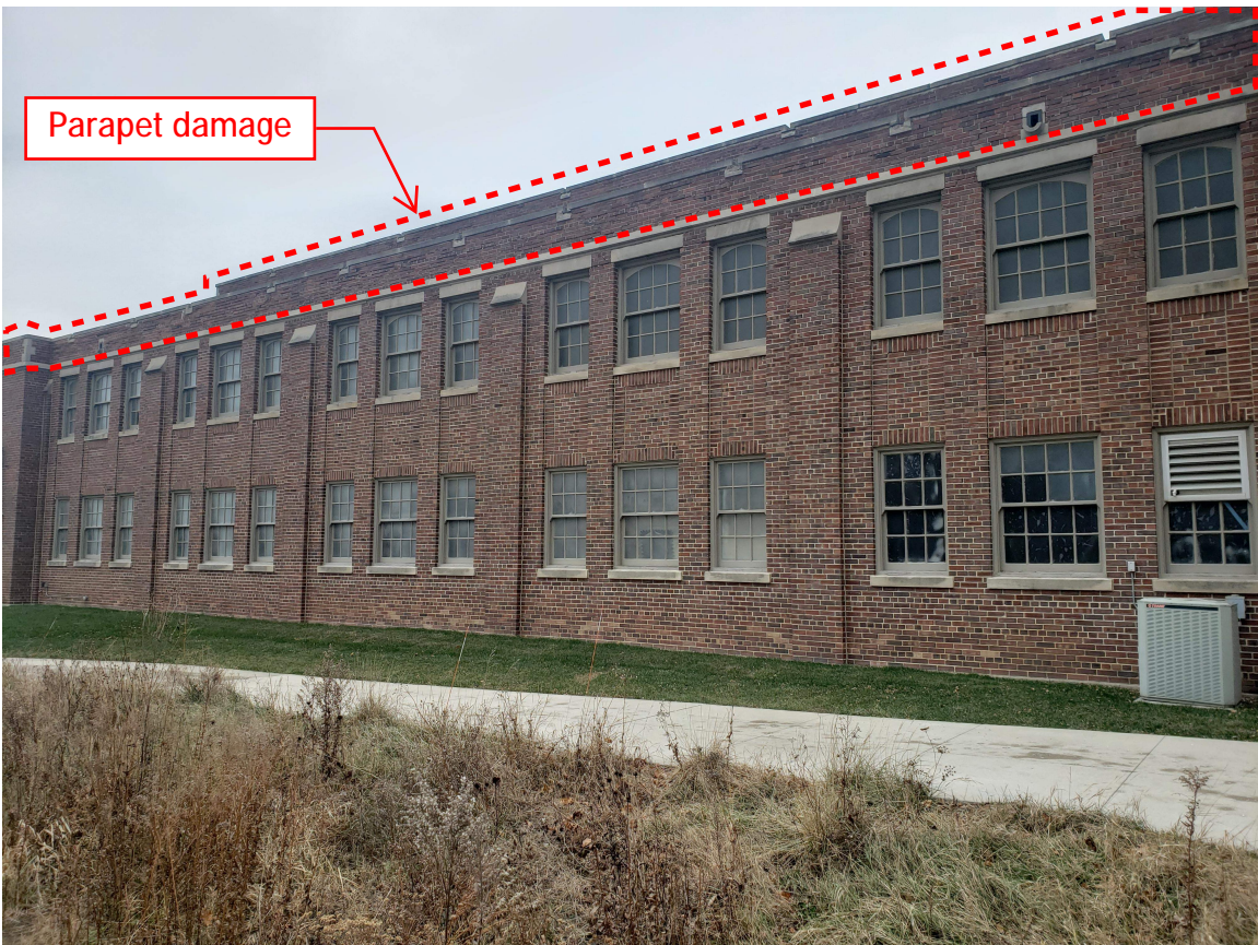
Photo 9 - East (central portion) at Gymnasium
