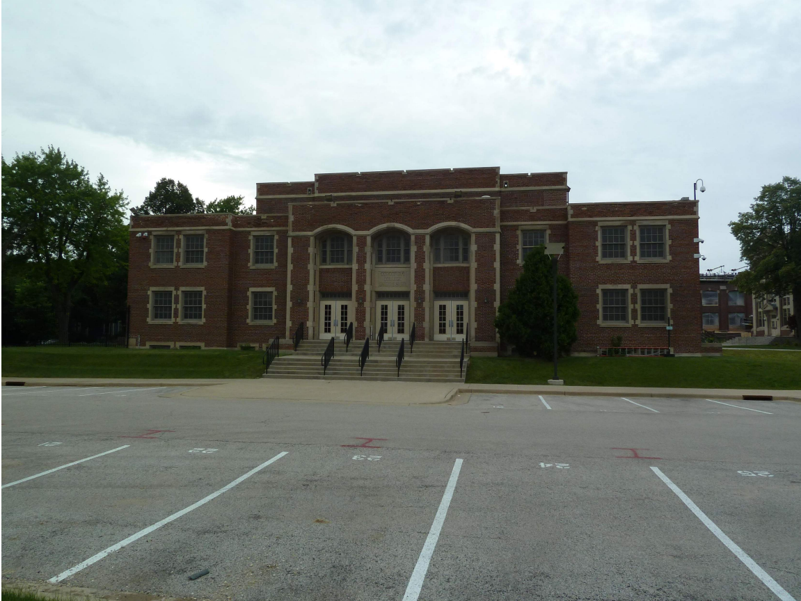
Photo 2 - South Overall at Gymnasium
