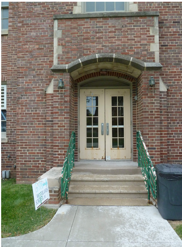
Photo 11 - East Entry (northern portion) at Gymnasium
