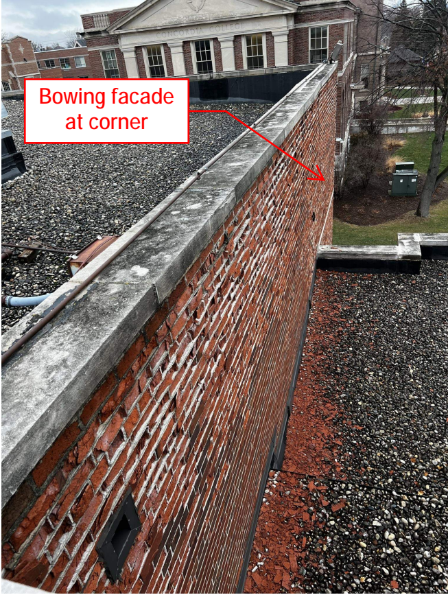
Photo 33 - South elevation bowing and brick damage at Pool Addition
