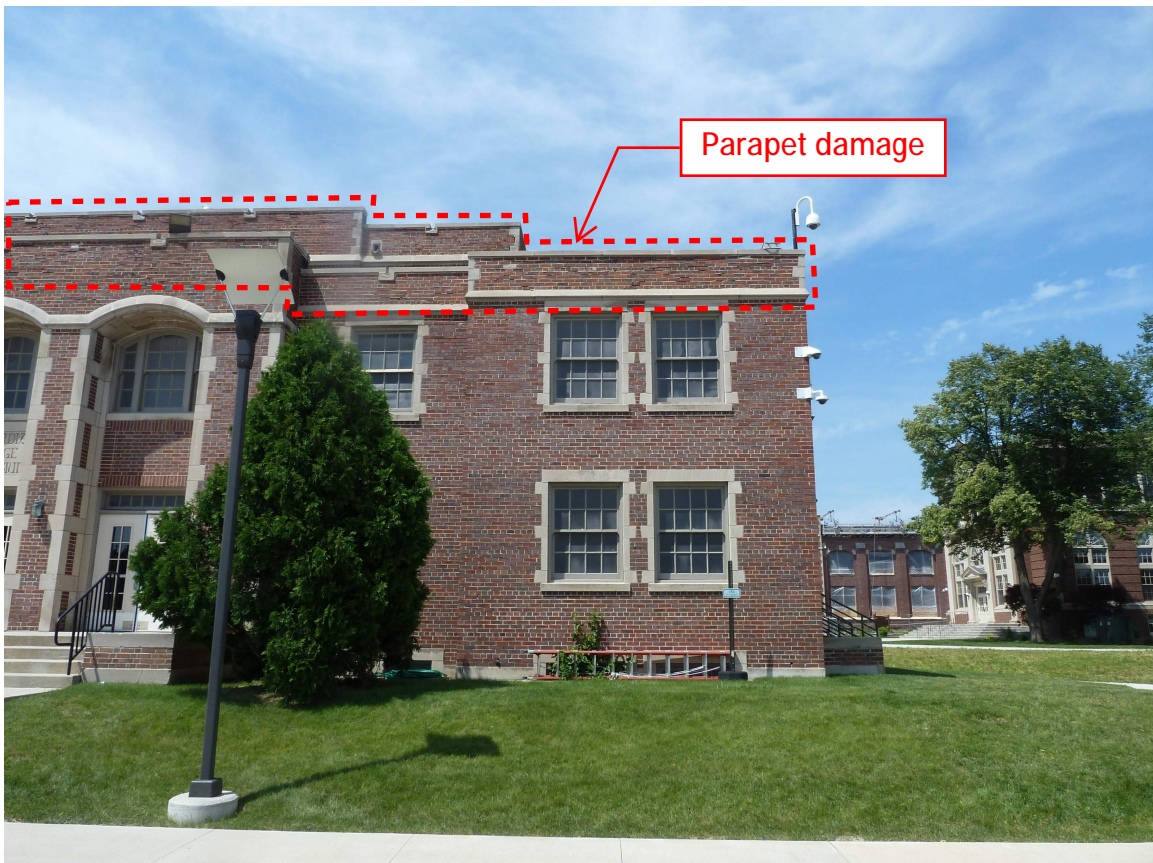
Photo 5 - South (eastern portion) at Gymnasium
