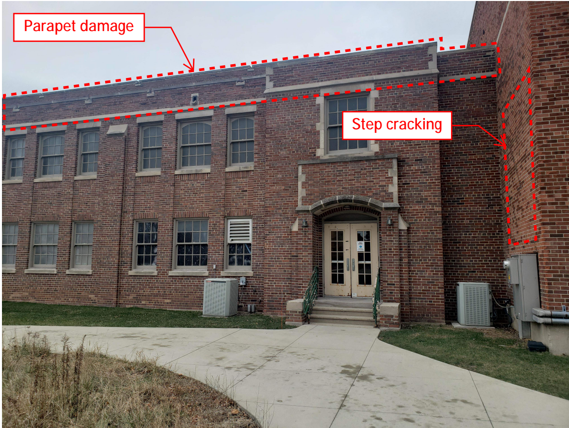
Photo 10 - East (northern portion) at Gymnasium
