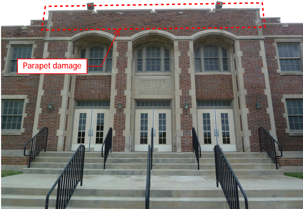
Photo 4 - South (central portion) at Gymnasium
