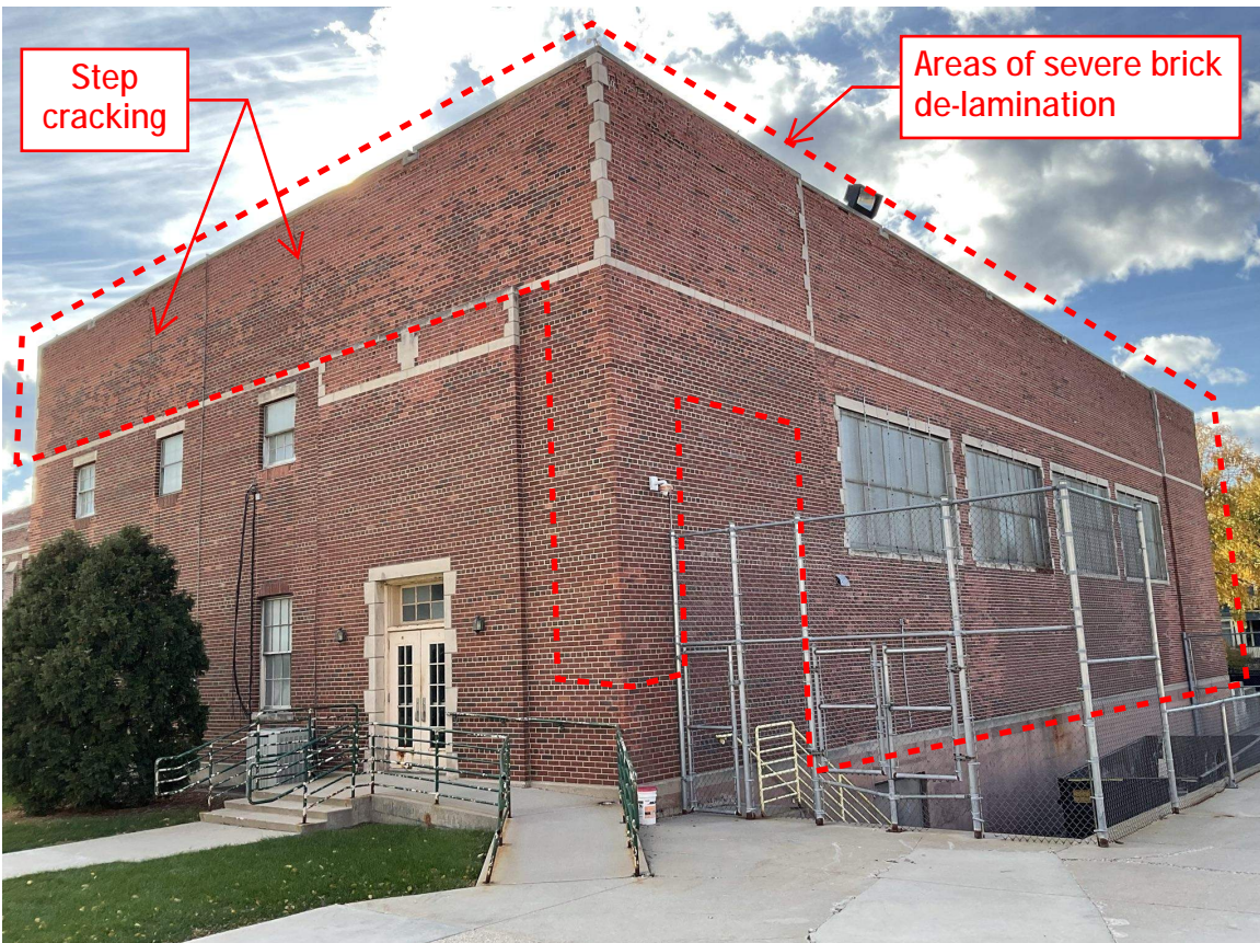
Photo 22 - North-east corner at Pool Addition
