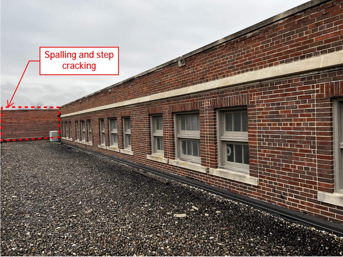
Photo 16 - Upper Windows at Gymnasium
