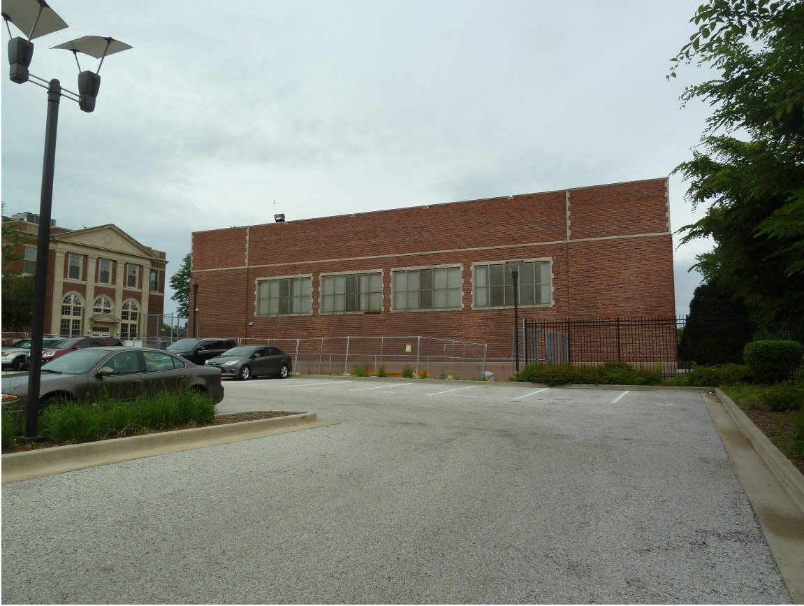
Photo 21 - North Overall at Pool Addition
