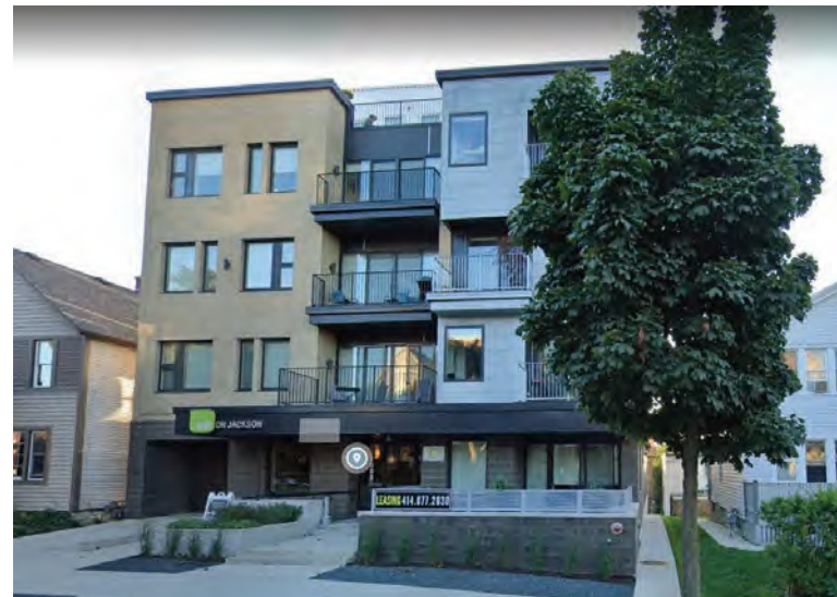
▲ Examples of recent, mid-scale, high quality redevelopment and development in Bay View and in other Wisconsin neighborhoods. (Marty Peters, top; Google, bottom)
