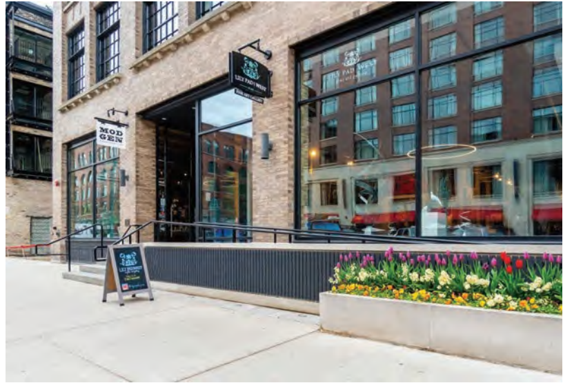
▲ Storefront with ample glazing, attractive signage, and plantings. Note the accessibility ramp. Source: Hyler Media
