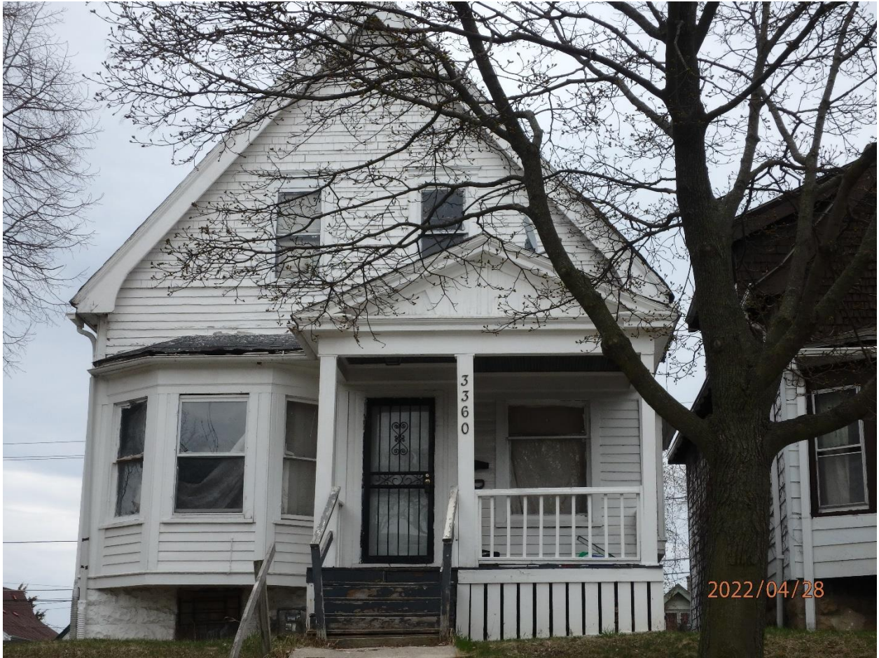
3360 North 21 st Street
