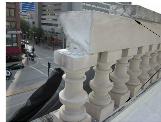
BALUSTRADE SILL/BASE CONDITION, TYP.
