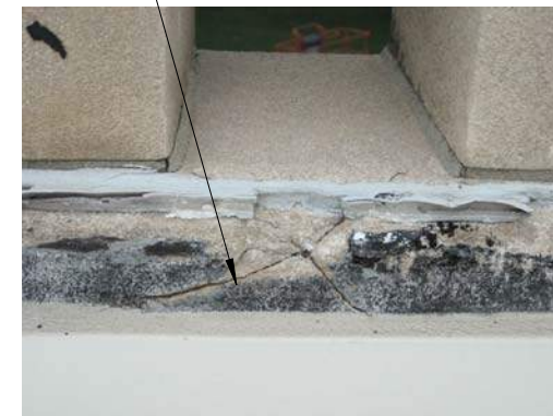
BALUSTRADE SILL/BASE CONDITION, TYP.
