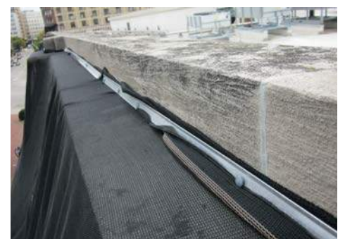
SAFETY NETTING ROLLED BACK, TEMPORARILY, TO SURVEY EXPOSED PARAPET FROM ROOF-SIDE.
