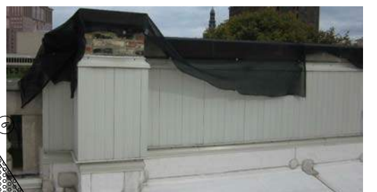
EXISTING SAFETY NETTING AT SOLID PARAPET, ROOF-SIDE.
