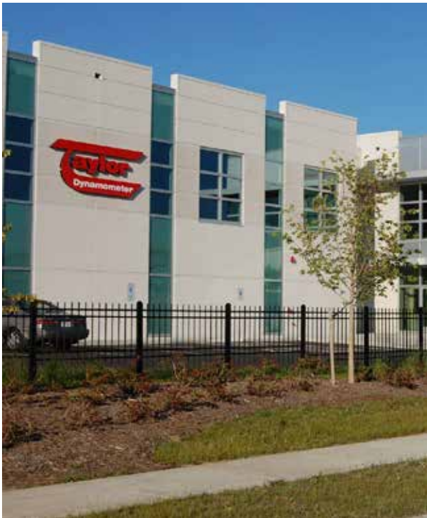
Taylor Dynamometer is a local company that has resulted from innovative entrepreneurship. (Source: Department of City Development / Planning)
