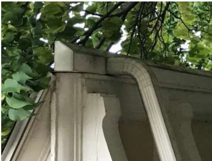
Closeup of existing gutter
