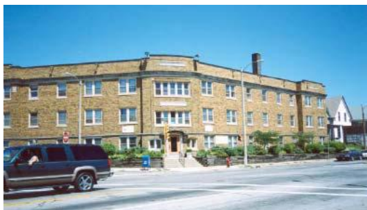
Existing UMCS Building
